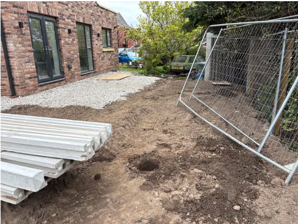
Plot 2 Garden: imported green field topsoil placed in garden
