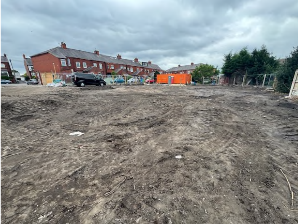
Plots 1 - 4 Gardens: Contaminated topsoil removed, natural subsoil exposed
