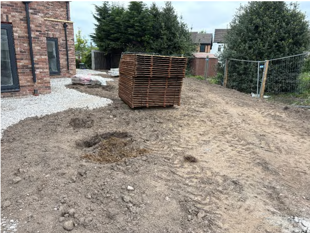
Plot 4 Garden: imported green field topsoil placed in garden
