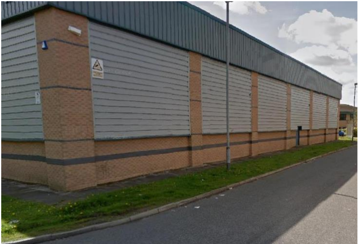
(Figure 9: This is the location of a previous approved application (Ref: 23/00071/TELE) that falls outside of the search area for this application but still carries valid precedent in sitting telecoms equipment within a business/retail park. Source: Planning Portal)
