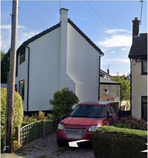
Streetview Photo-Existing Side Elevation
