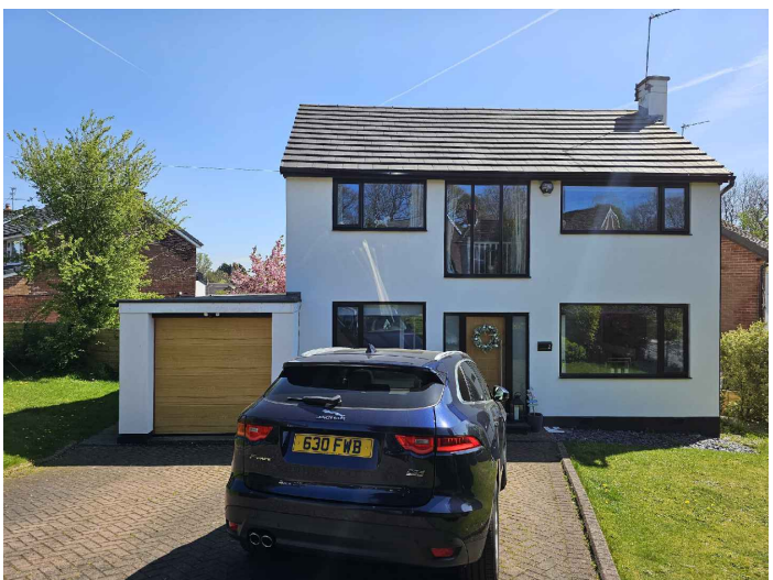
Site Photo-Existing Front Elevation
