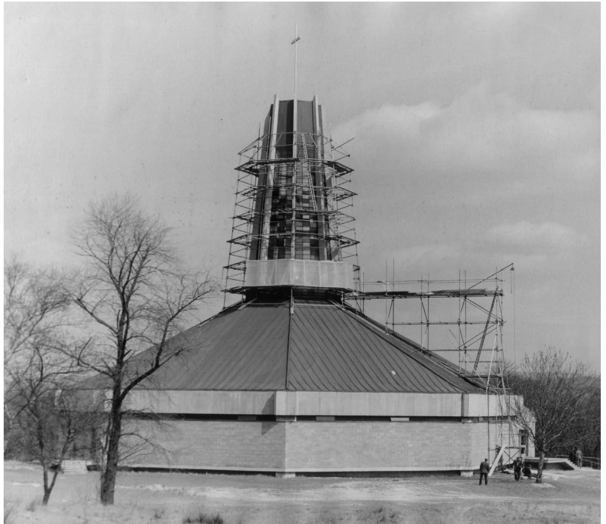
Figure 4.1 The Chapel during construction (Source: Rochdale Archives)
