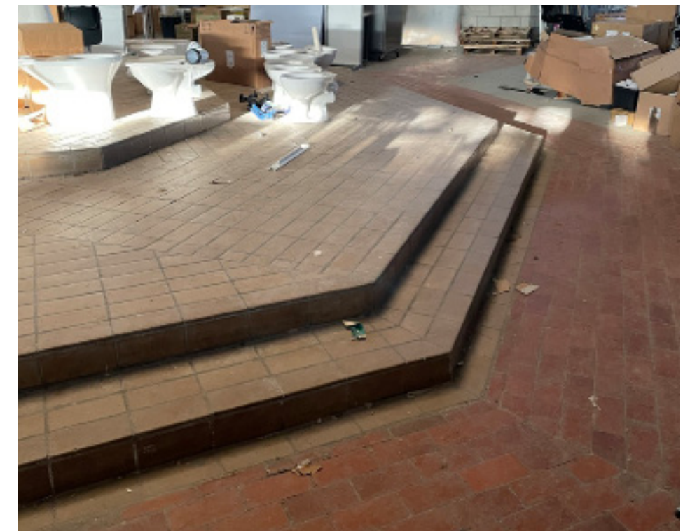
6 Central steps in the hall.
