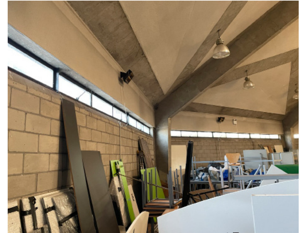
3 High level glazing above exposed blockwork walls.
