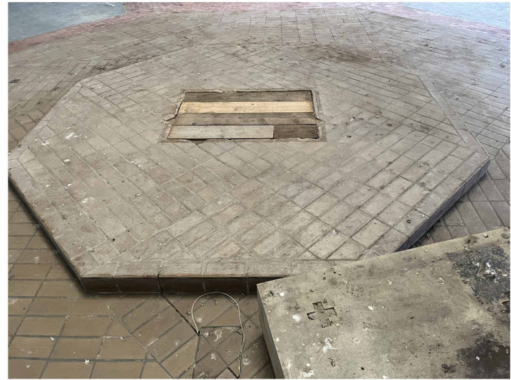
PHOTOGRAPH OF ORIGINAL STONE BLOCKWORK FORMING BASE OF ALTAR
