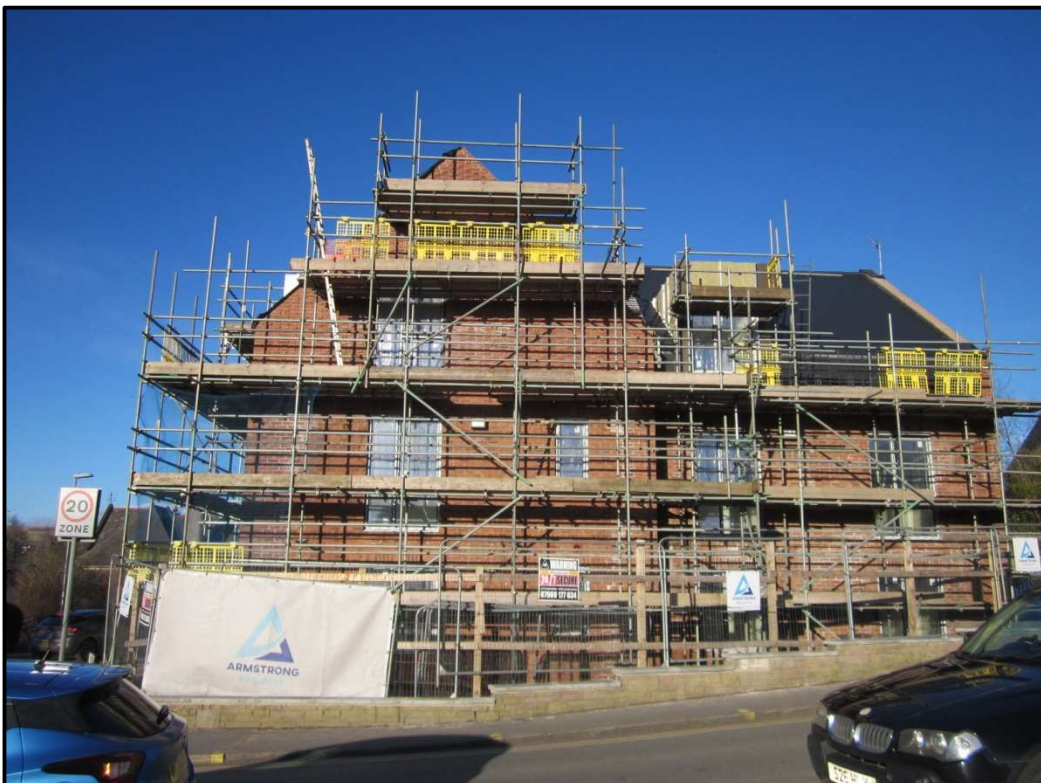
Photograph 1. Former Smithy Bridge public house (looking North)
