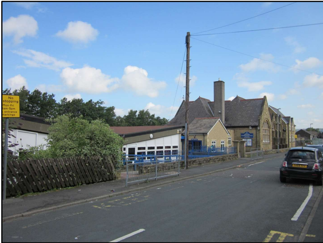
Photograph 2. Bridgenorth Drive and the Smithy Bridge Foundation Primary School to the North West of the proposed development
