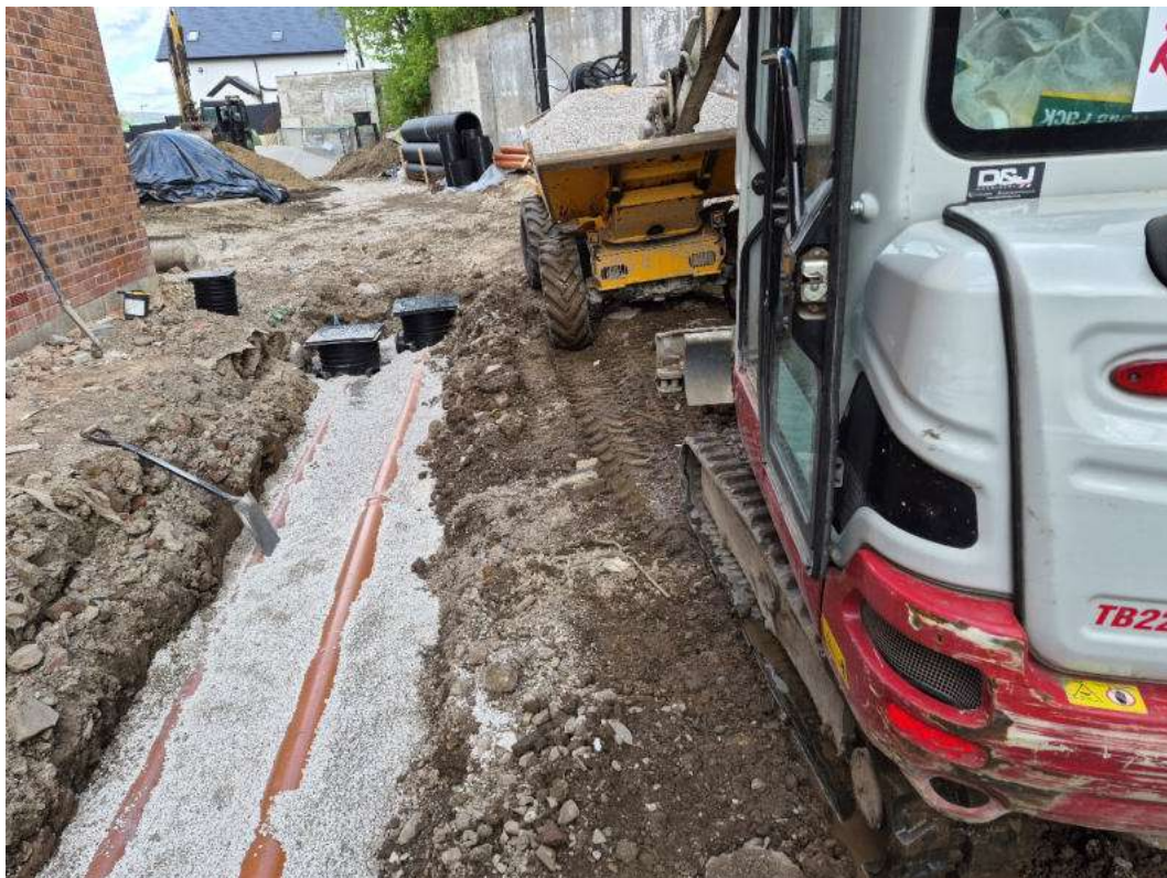
Photograph 14: Installation of drainage along the side of the building – 6/5/2026
