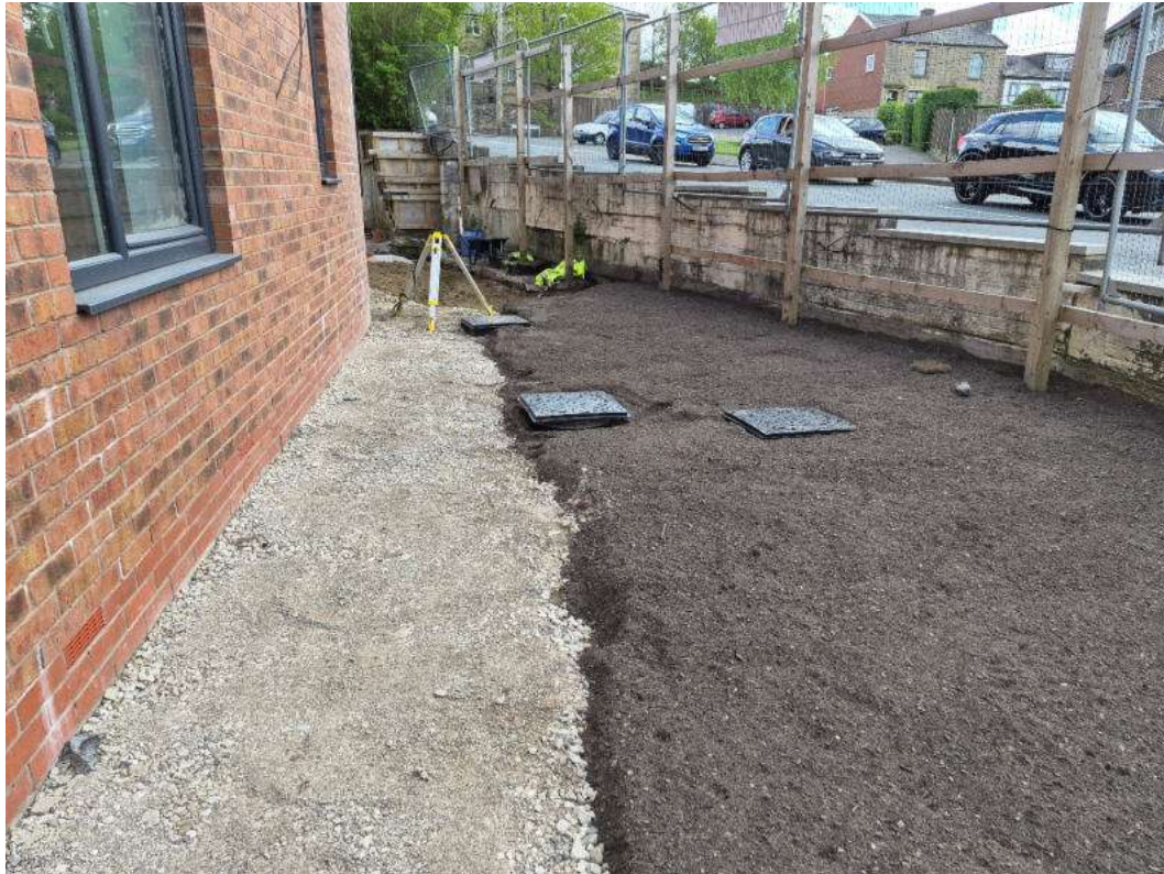
Photograph 13: Area of full subsoil and topsoil application to the front of the building along Smithybridge Road - 6/5/2026.
