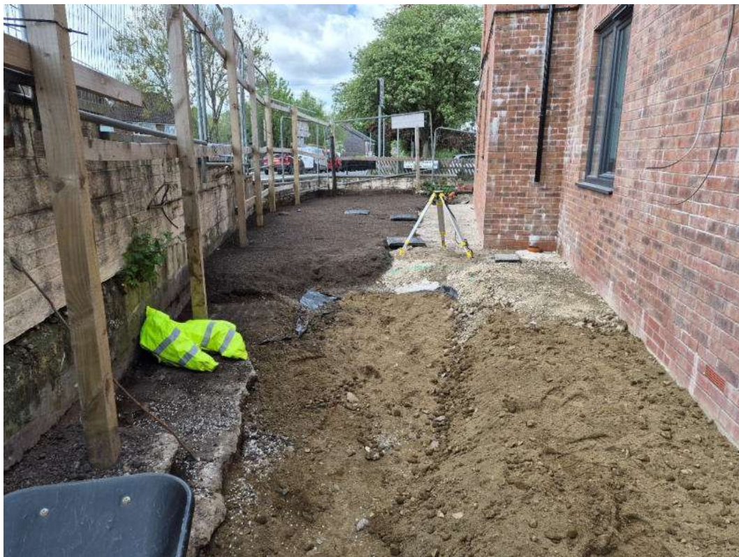
Photograph 10: Partial application of subsoil and topsoil to the front of the building along Smithybridge Road - 6/5/2026.
