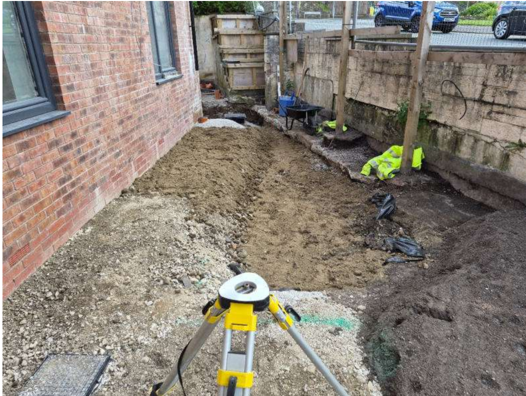
Photograph 11: Partial application of subsoil and topsoil to the front of the building along Smithybridge Road - 6/5/2026.
