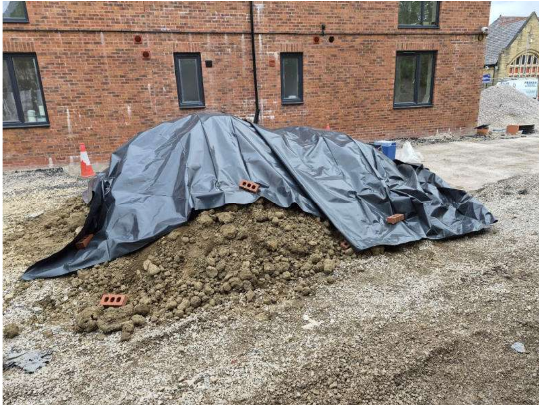
Photograph 3: Stockpile of imported subsoil - - 28/04/2026
