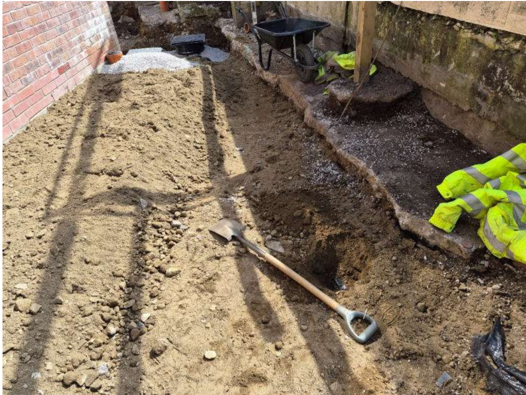
Photograph 17: Validation Pit 3, located in area with subsoil cover but prior to application of topsoil – 6/5/2026.
