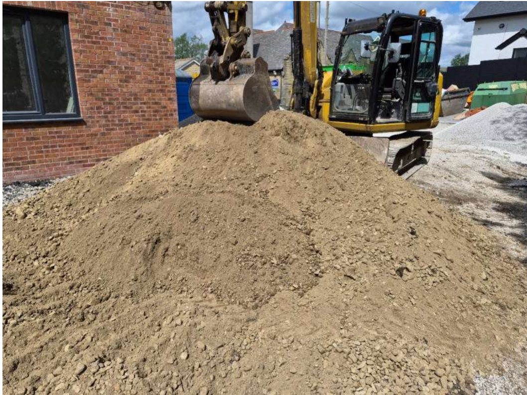
Photograph 19: Stockpile of subsoil tested during previous validation visit – 6/5/2026.
