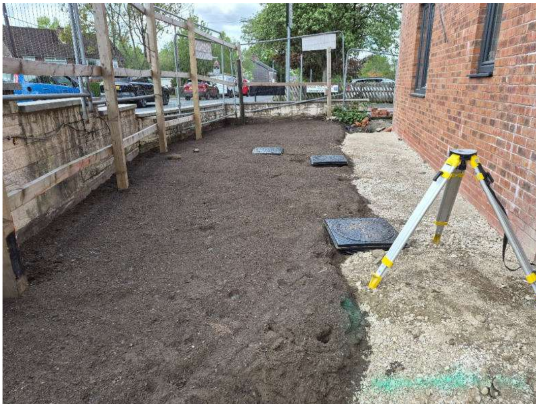
Photograph 12: Area of full subsoil and topsoil application to the front of the building along Smithybridge Road - 6/5/2026.
