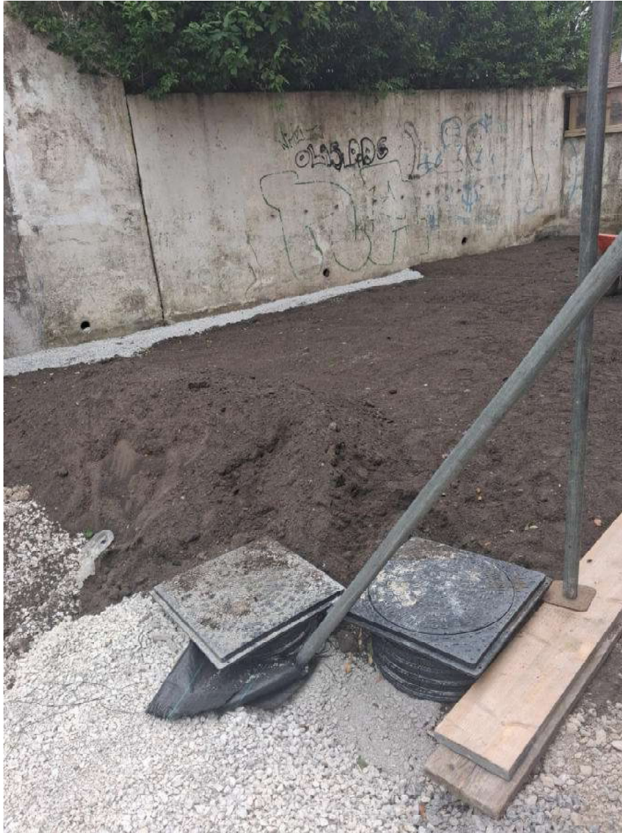
Photograph 21: Final Application of clean cover to landscaped area to the side of the building. Photographs supplied by the contractor on the 1/6/2026.
