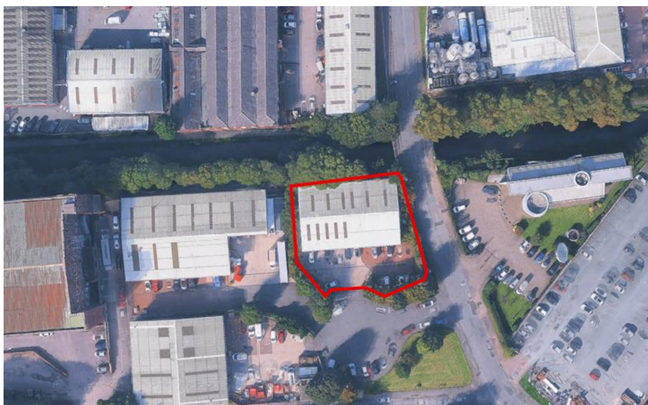
Fig 2.1: Aerial view of the site (outlined in red).
