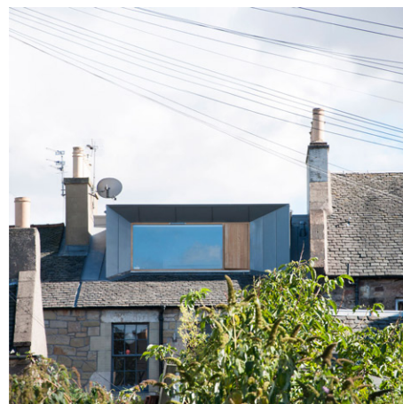
Figures 2 & 3: Detail views of zinc cladding, timber window surround, and low-profile form within the roofscape. Architect: Konishi Gaffney. Photography: Alan Craigie. Source: Dezeen.
