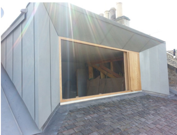
Figures 2 & 3: Detail views of zinc cladding, timber window surround, and low-profile form within the roofscape. Architect: Konishi Gaffney. Photography: Alan Craigie. Source: Dezeen.
