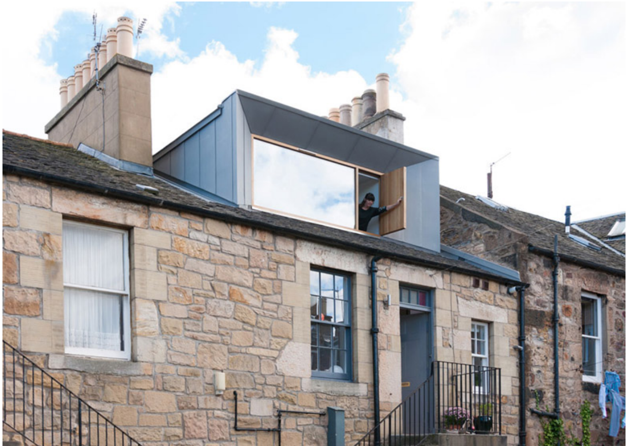
Figure 1: Regent Street Dormer, Edinburgh. Zinc-clad flat roof dormer to Victorian stone terrace. Architect: Konishi Gaffney. Photography: Alan Craigie. Source: Dezeen.
