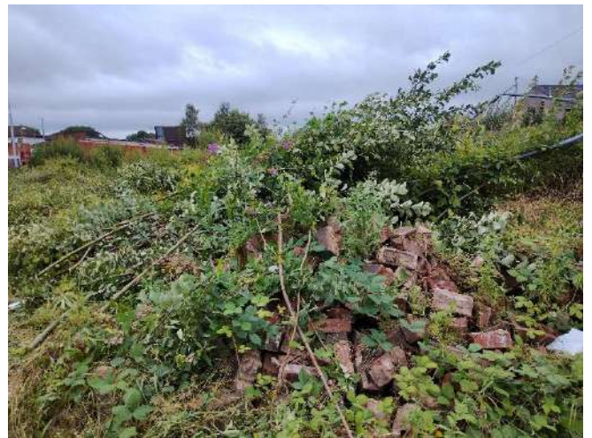
Figure 2 – Mound of bricks and demolition material in the north eastern site section.
