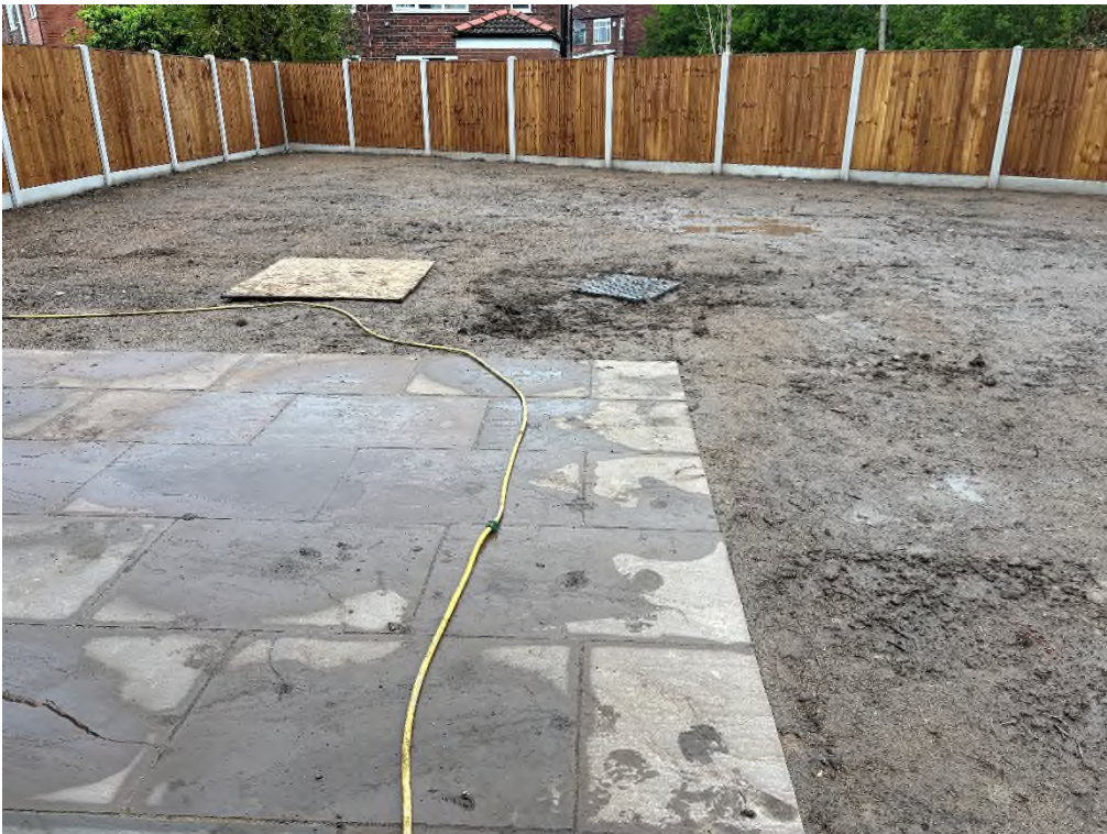
Plot 8 Garden: imported green field topsoil placed in garden
