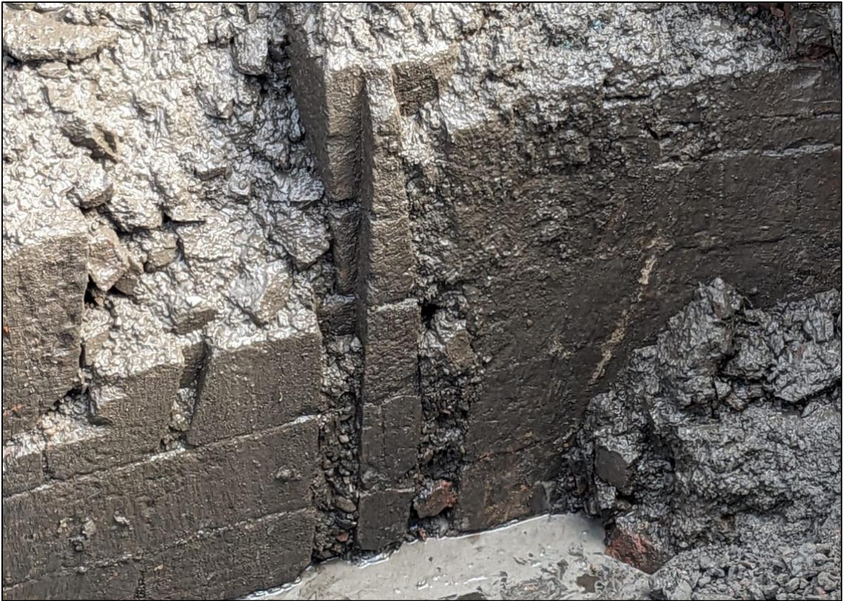
Plate 14: sluice gate housing in wall 14, looking east
