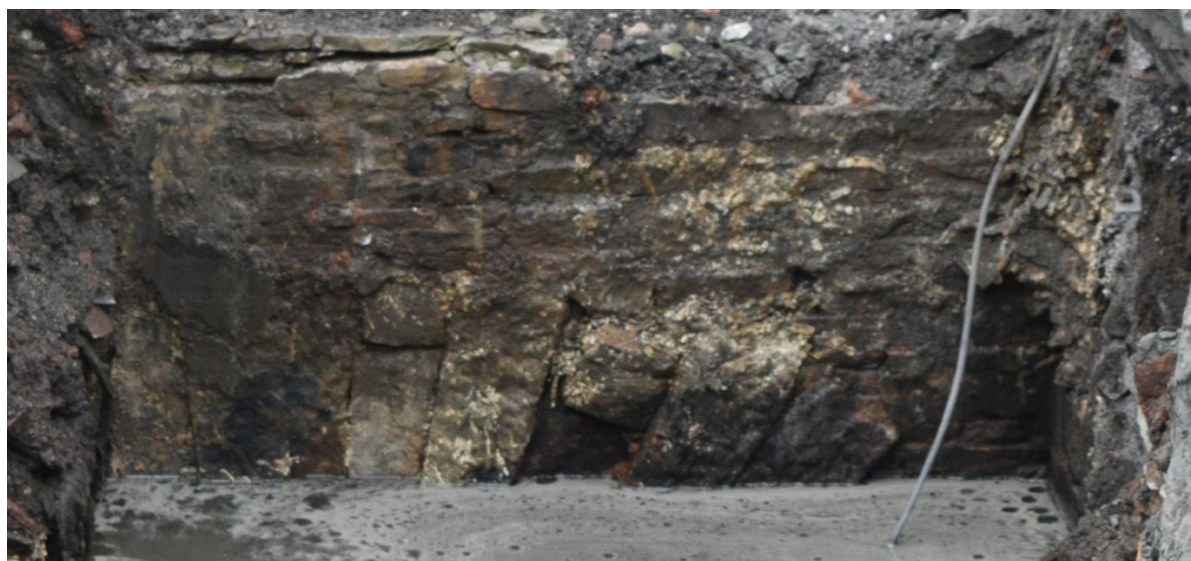
Plate 11: Voussoirs in wall 13, looking northwest
