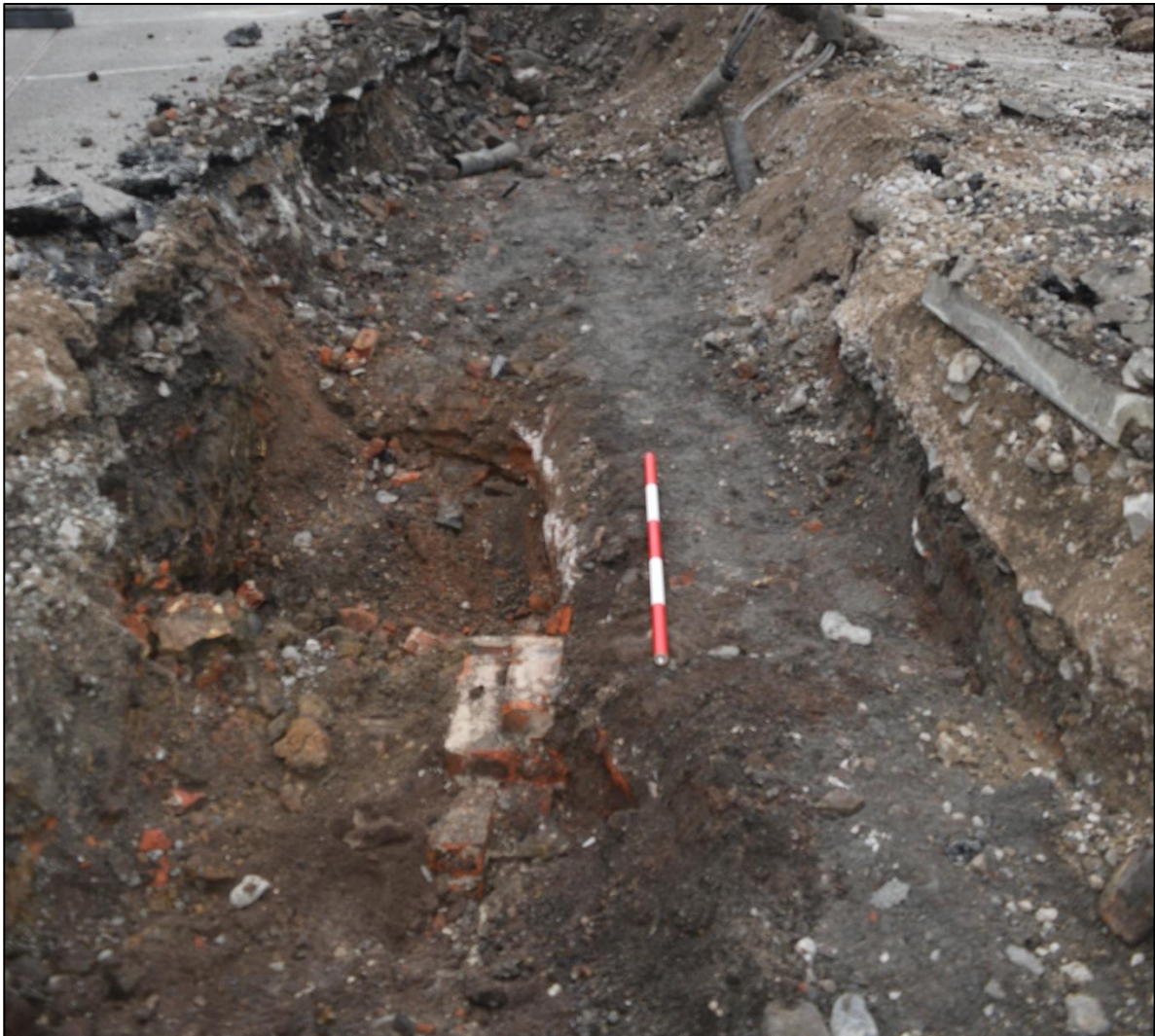
Plate 7: Ground beams in trench 2, looking east
