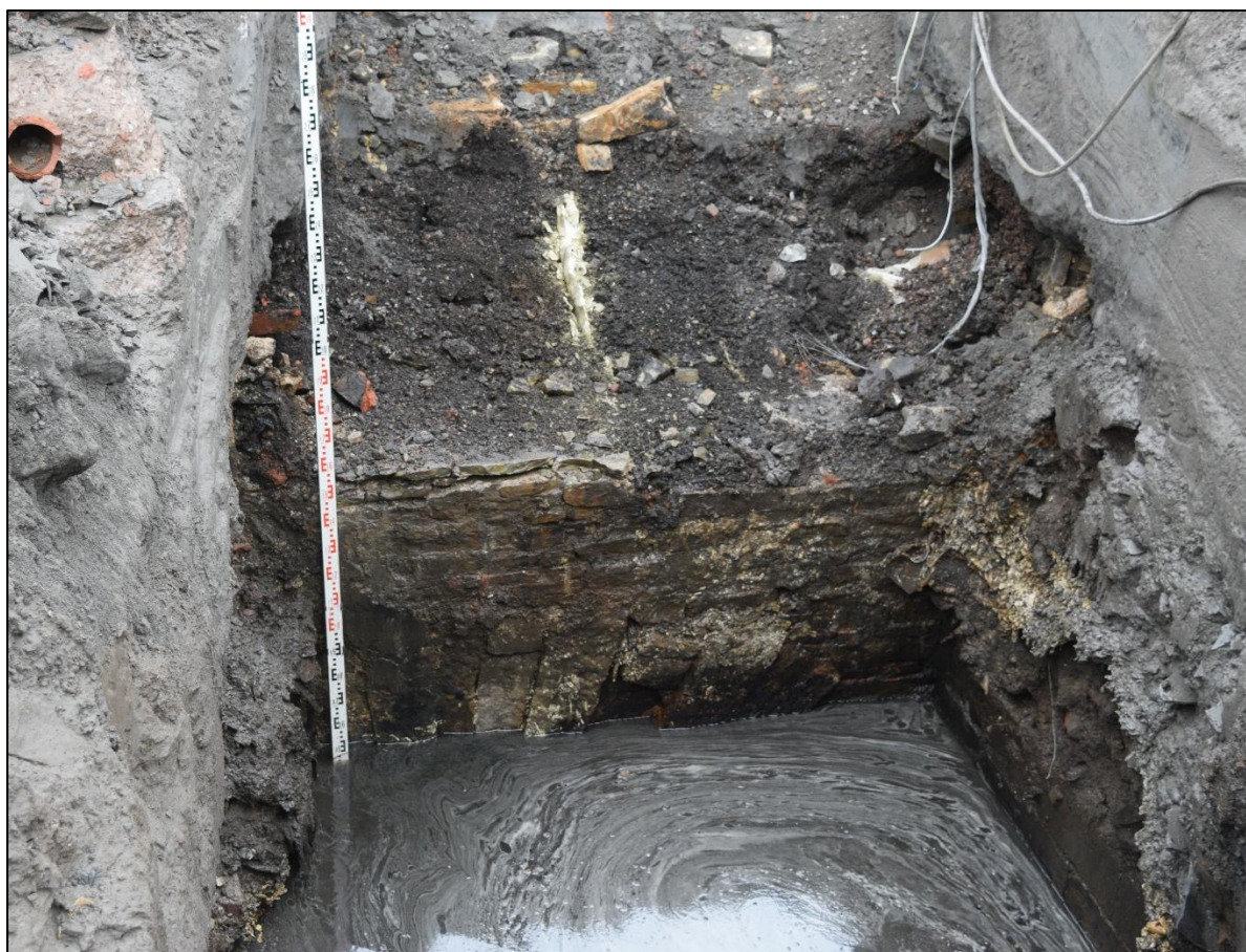
Plate 10: Walls 12, 13 and 14, looking northwest
