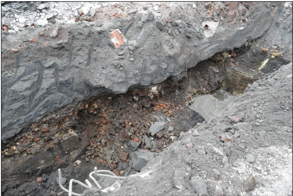
Plate 16: Overburden and fly ash capping, looking west
