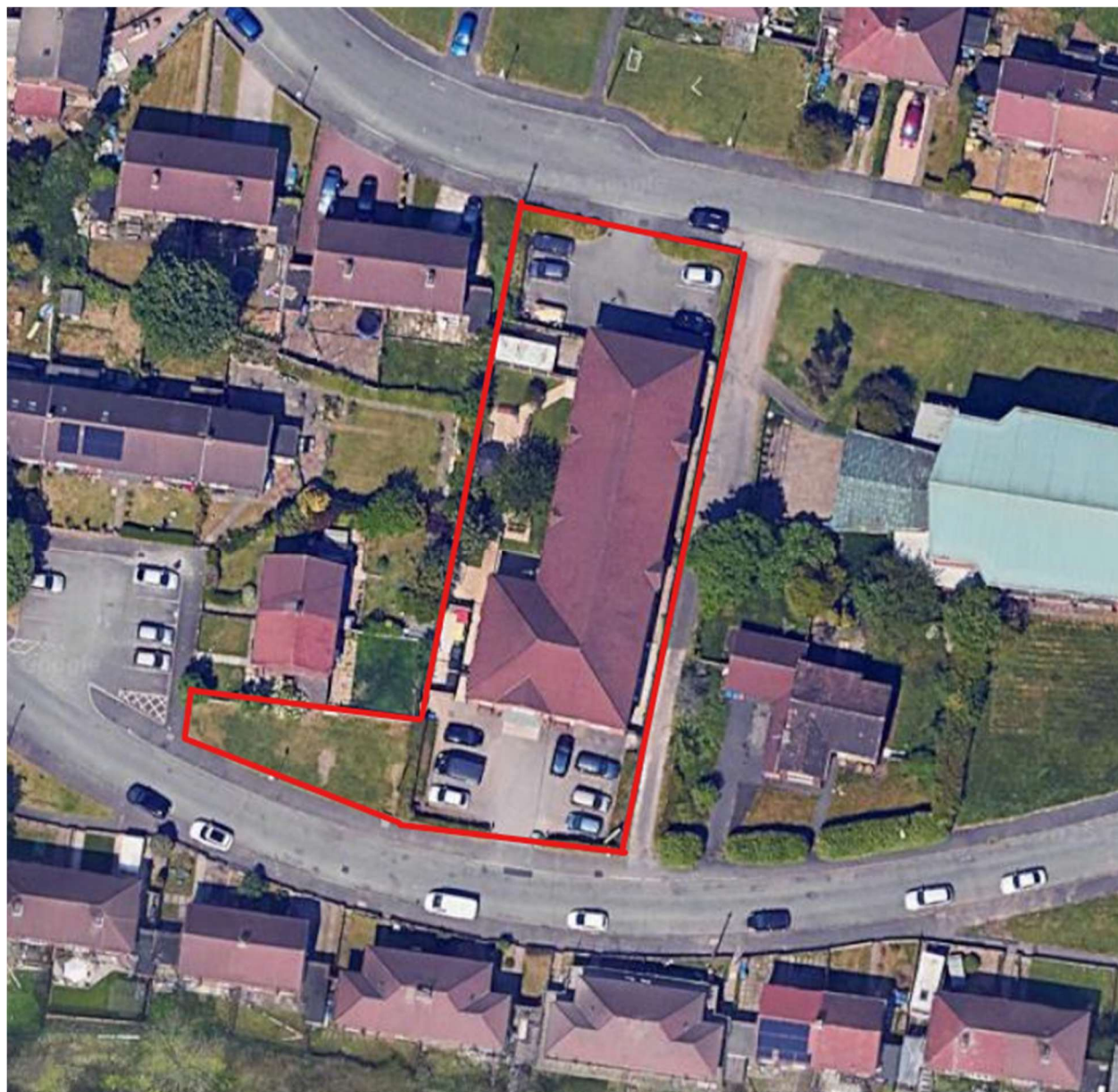
Figure 1 Aerial view of Application Site in red.
