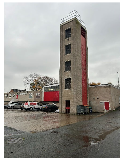
Rear view of the existing fire station
