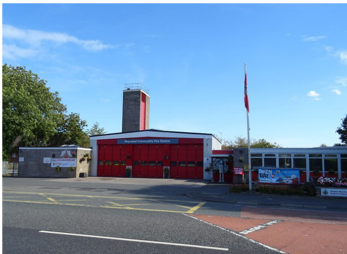
Front view of the existing fire station
