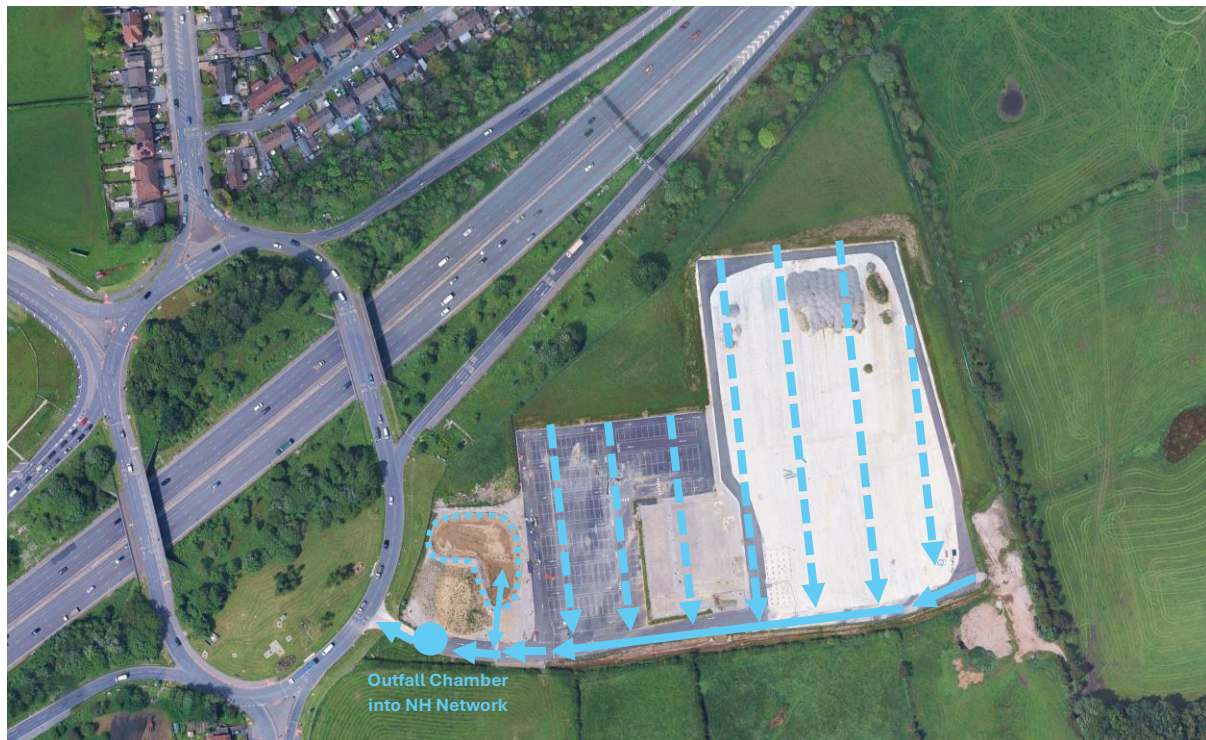
Figure 3: Temporary Site Compound constructed in 2023 and current as-built site condition
