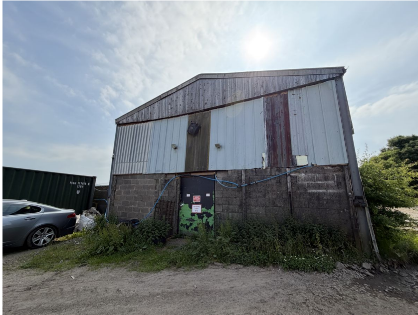
Figure 1: The application building, set within its existing fenced yard and the surrounding Green Belt landscape.
