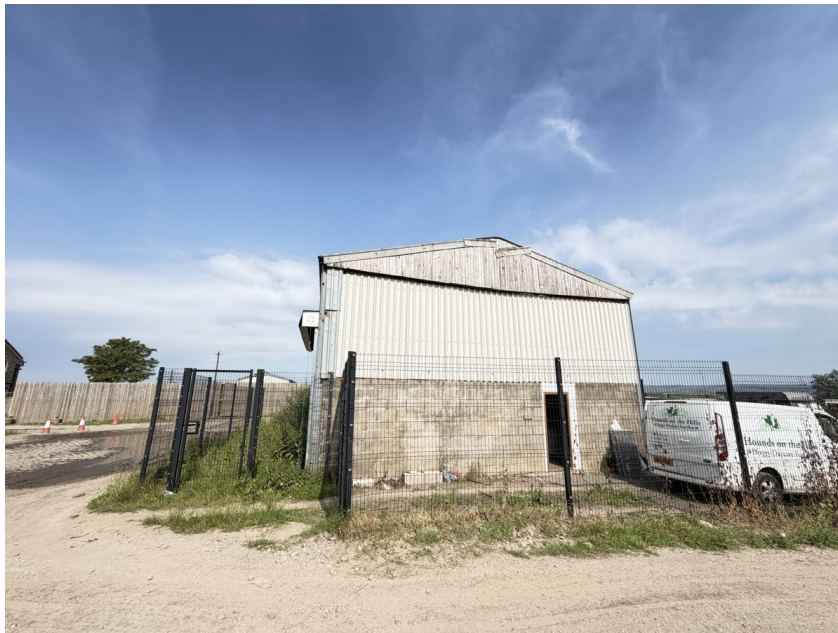
Figure 2: Existing barn, gable elevation, showing the existing entrance door and boundary fence line.
