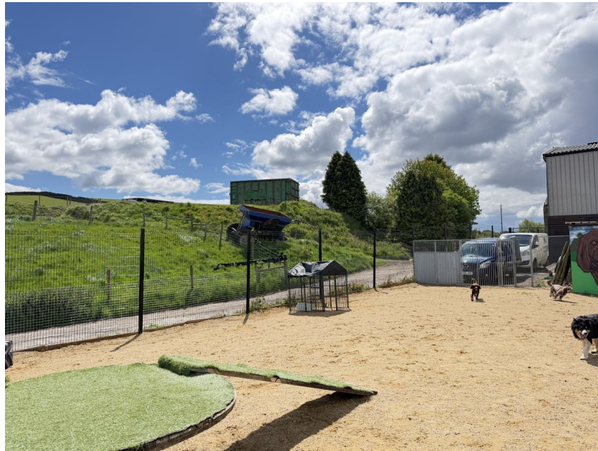
Figure 4: Existing mesh panel fencing and gated yard access, of the type proposed for the new fence link.
