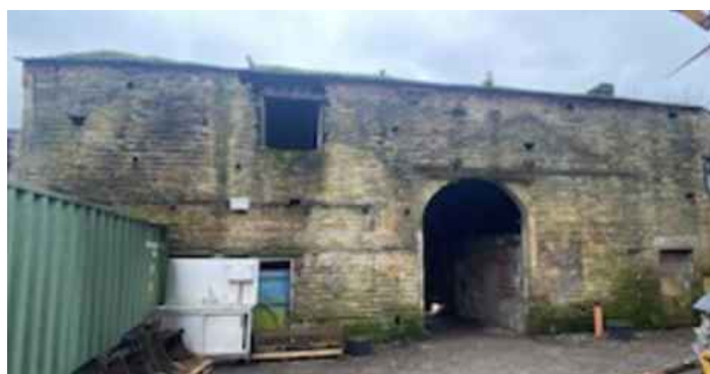
Existing Rear Elevation (photo)
