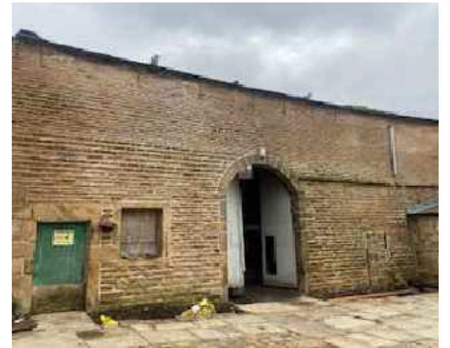
Existing Front Elevation (photo)
