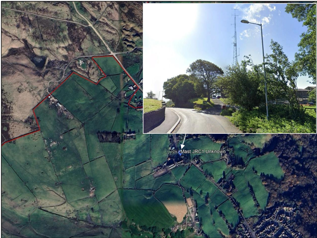
Figure 6 Aerial and Streetview imagery of the JRC mast
