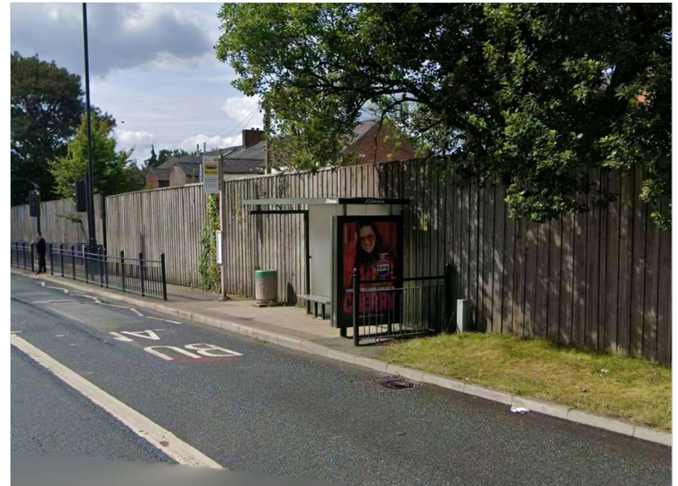
Southbound view of existing shelter
