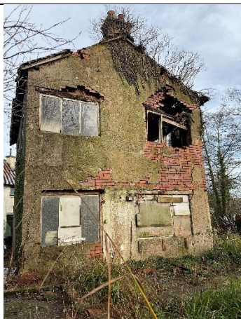
Photo 7: Unannotated images of southern face.
