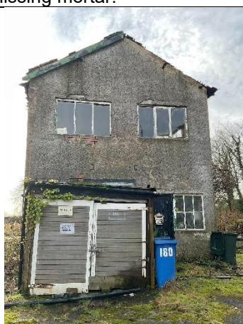
Photo 5: Unannotated images of northern face.
