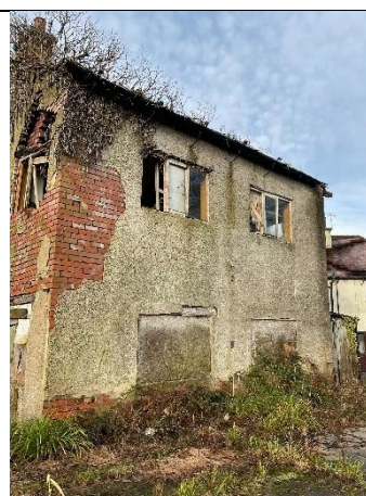
Photo 6: Unannotated images of eastern face.
