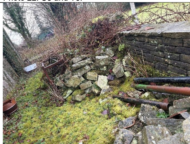
Photo 24: S2 with piles of rocks.
