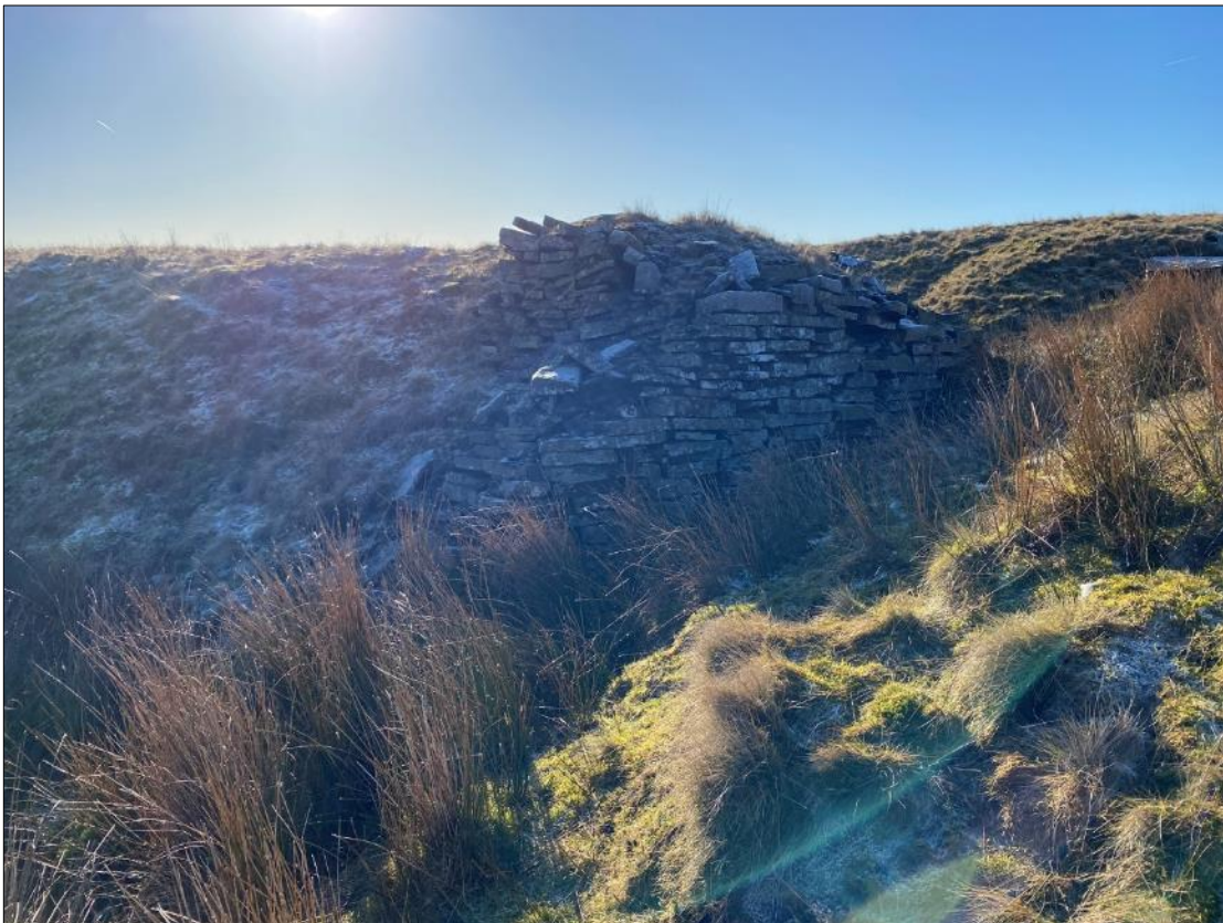
Plate 76: Revetment wall at end of spoil tip, Ding Quarry.
