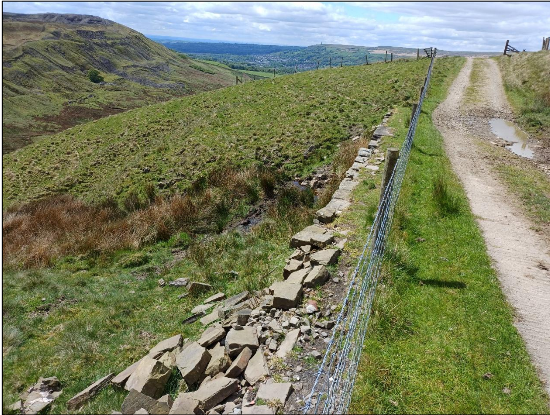
Plate 89: View west of detail of structure along section of route which crosses a brook
