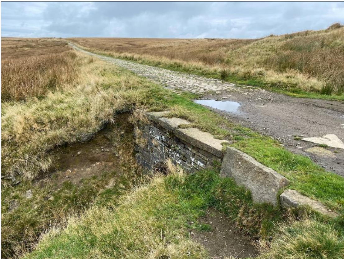
Plate 18: Looking north along a section of Rooley Moor Road (Asset 828) at Hamer Hill with a stone bridge (Asset 923).
