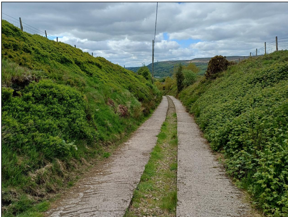
Plate 100: View southwest along Gincroft Lane Street
