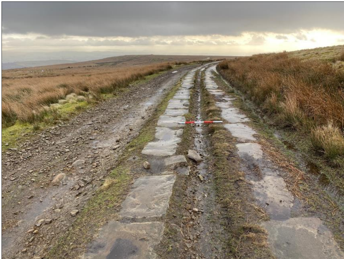
Plate 70: Condition of Rooley Moor Road at proposed crossing point of access track, just south of Asset 756.
