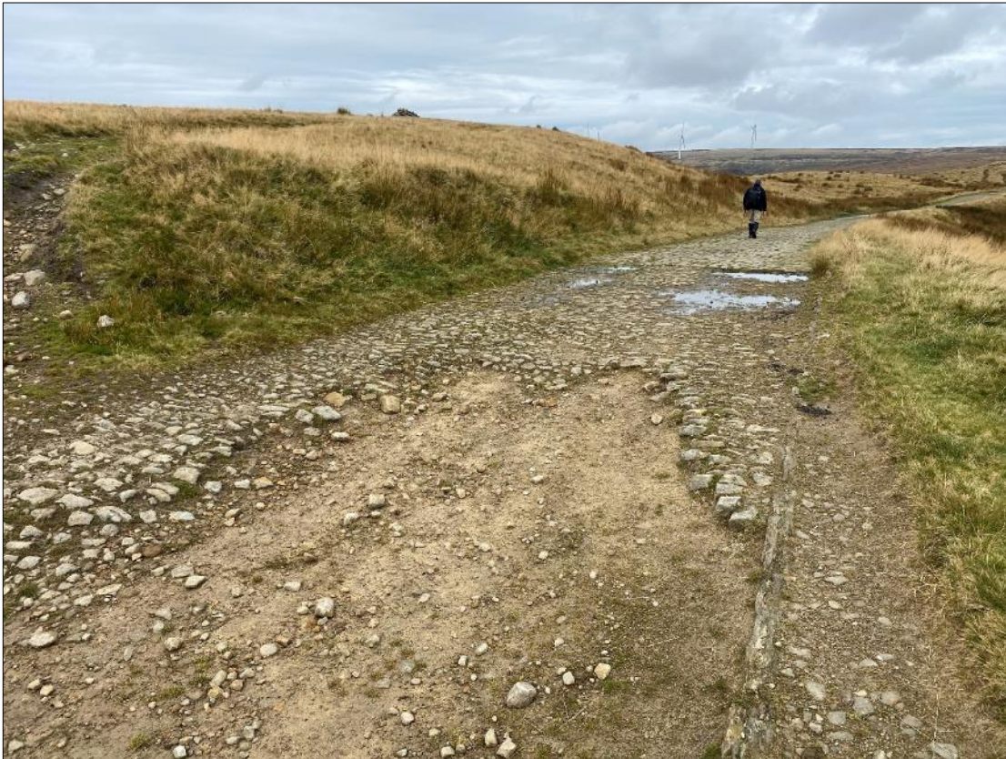
Plate 15: Looking NNW along a section of Rooley Moor Road (Asset 828) at Top of Pike.
