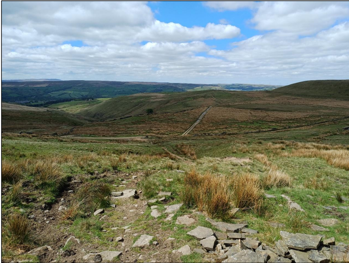
Plate 81: View west across eastern end of Alternate Grid Connection Route (Option C)
