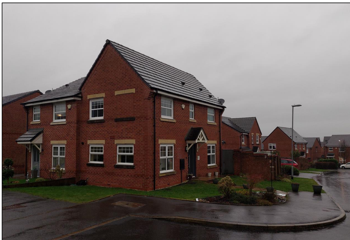
Nearby Corner Plot Development (Semi-Detached Building at South of Strawberry Close)
