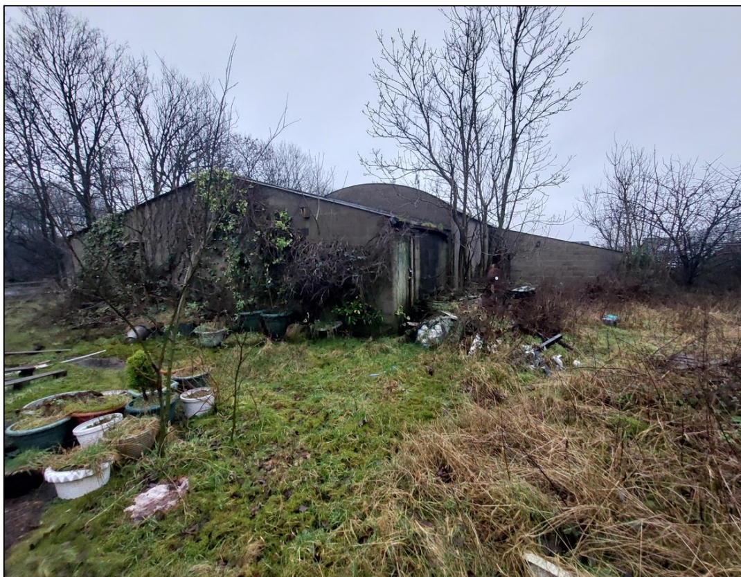
View of Dilapidated Former Agricultural Building (Facing West)
