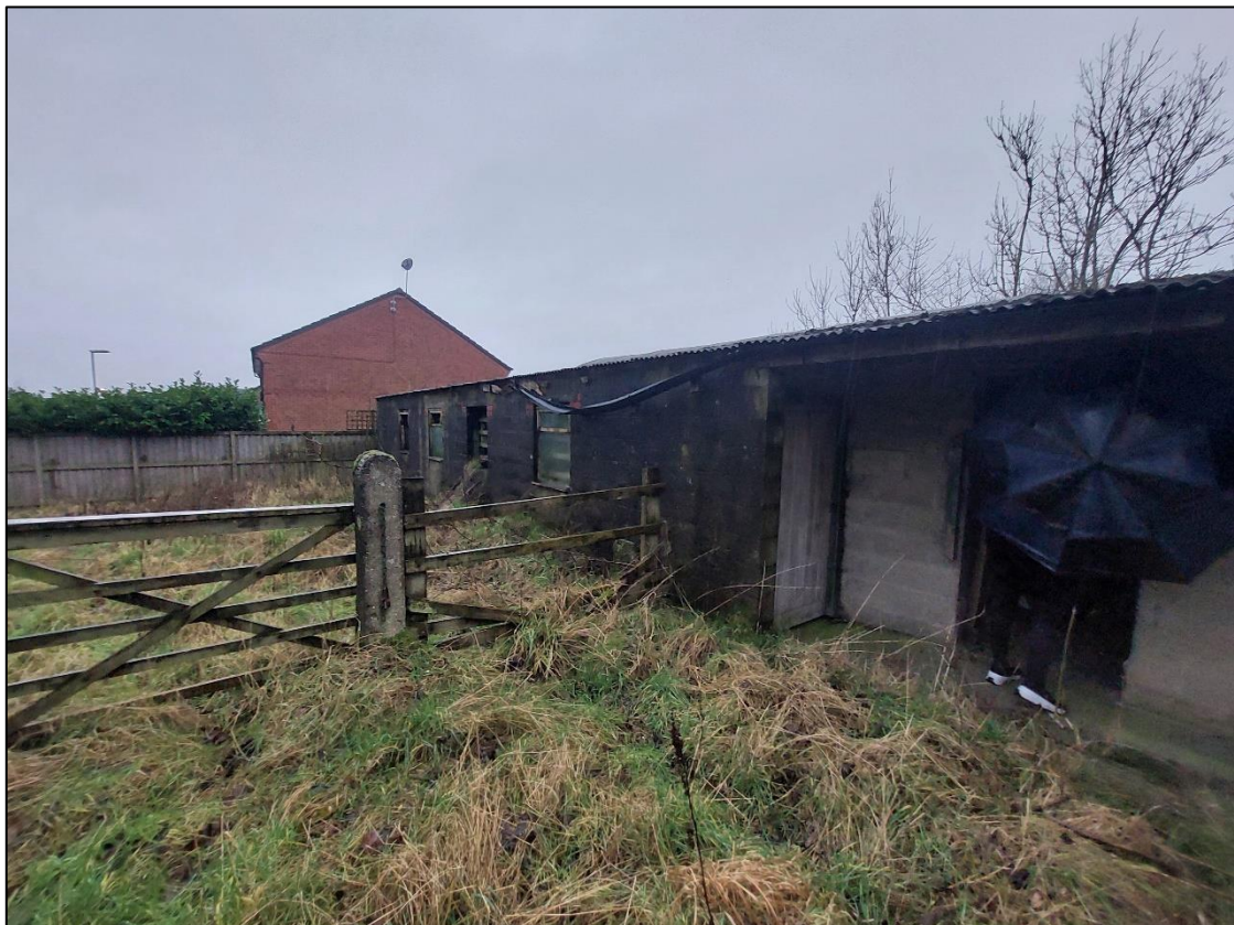
View of Dilapidated Former Agricultural Building (Facing North West)
