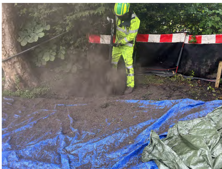
Image 1 – Air excavation in operation
