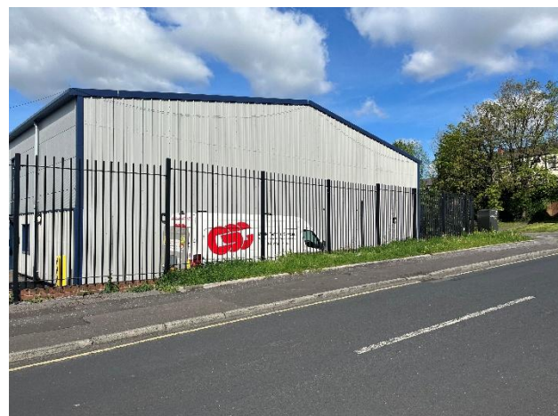
Fig 2.4 Image of site looking northwest on Primrose Street
