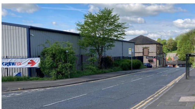
Fig 2.5 Image of installed fencing along Spotland Road boundary.
