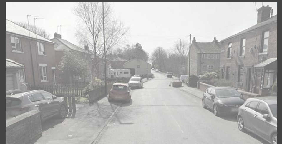
Ramsden Road looking westwards
