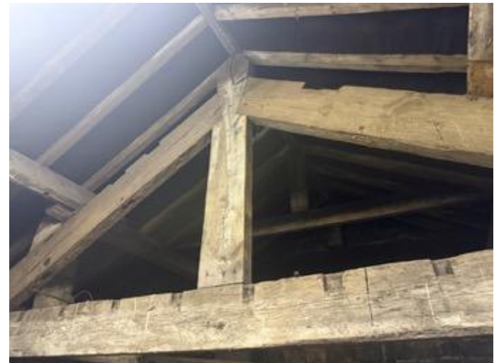
Internal area of B1
