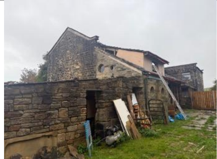
Northern elevation of B1
