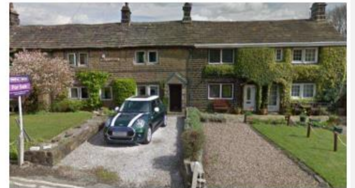
1 Lower Calderbrook Road (Front/Street Facing Elevation)
