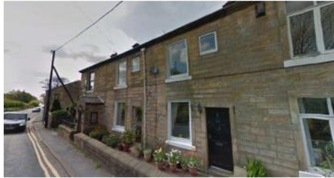
4-3 Handl Hall (Front/Street Facing Elevation)
