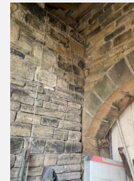
Joining of lean-to to barn
