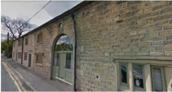
Handle Hall Farm (Front/Street Facing Elevation)
