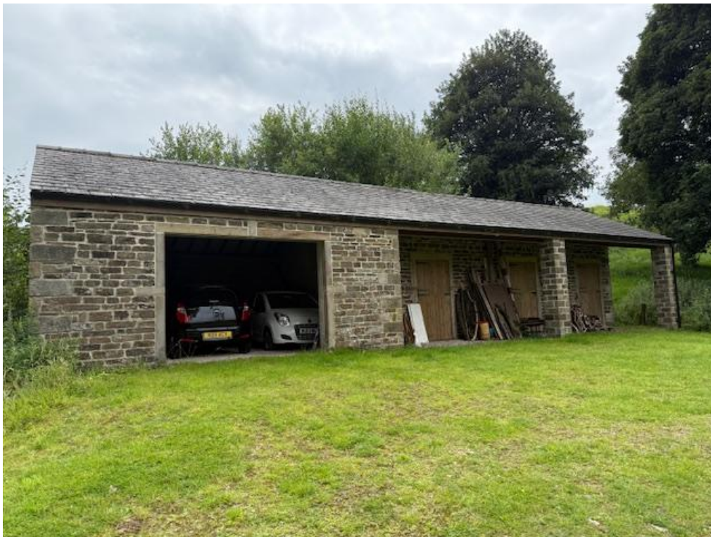
The application site
