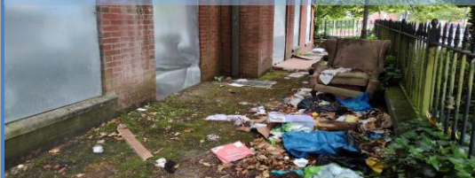
A view along the western end of the Yorkshire Street façade
