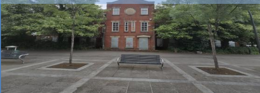
St James Place, number 168 Yorkshire Street and the pedestrianised space in front of the building
