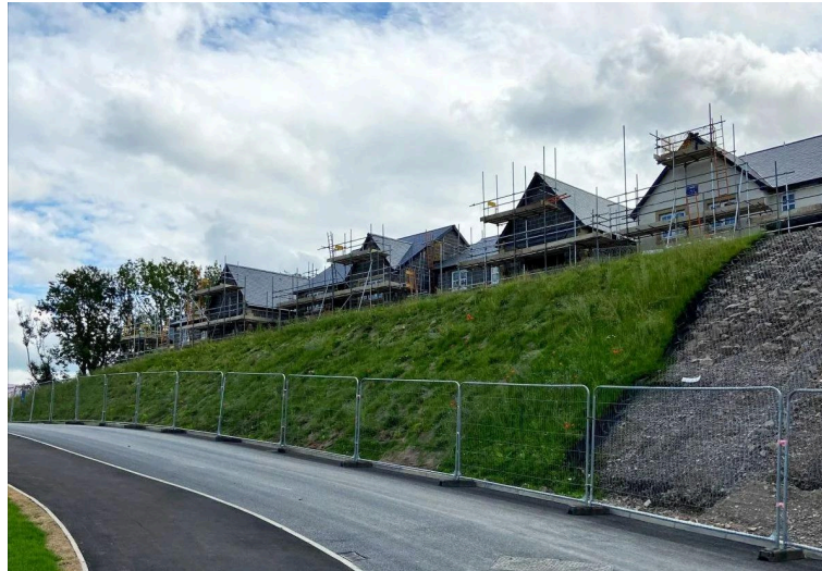
Engineered Reinforced Slope
