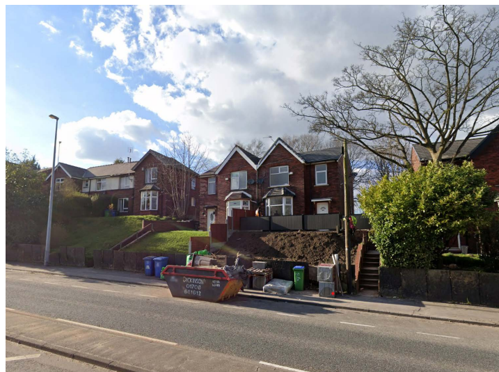
[02] STREET VIEW OF THE BUILT CONTEXT - ROCHDALE BYPASS
