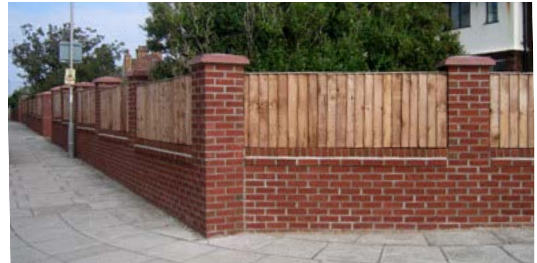
Example Brick Boundary Wall
