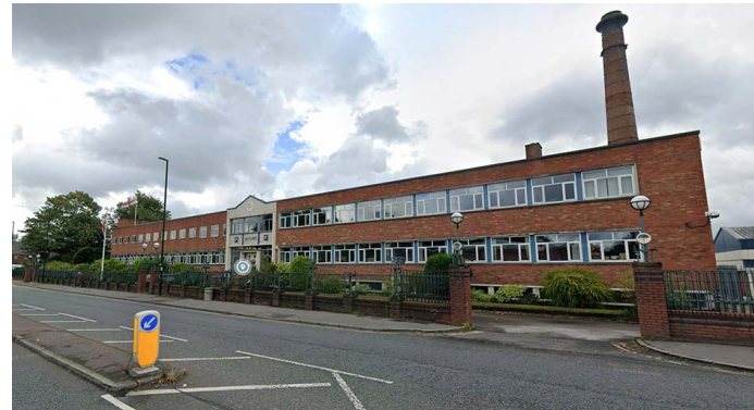
[03] 3D STREET VIEW OF THE BUILT CONTEXT- NORTH EAST
