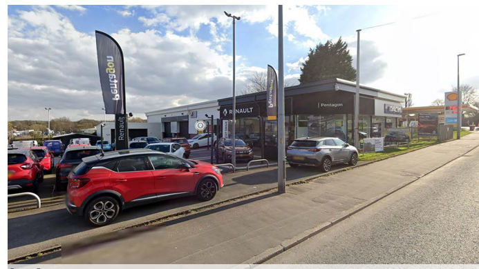
[04] 3D STREET VIEW OF THE BUILT CONTEXT- NORTH EAST
