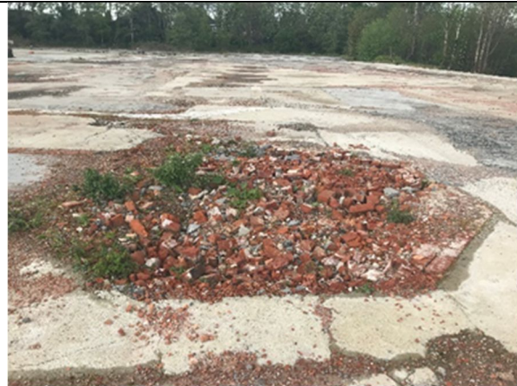
Photograph 9: Location of former chimney, central-east of site, facing north-east.
