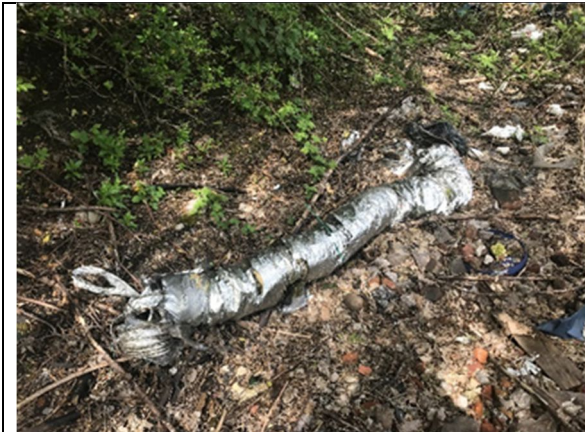
Photograph 7: Pipe with possible asbestos lagging, west of site.
