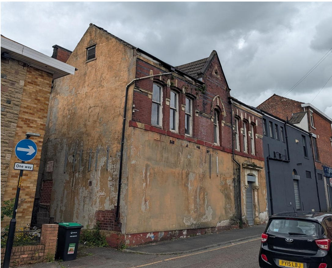
Figure 1: Existing Bethel Street frontage and side access.
