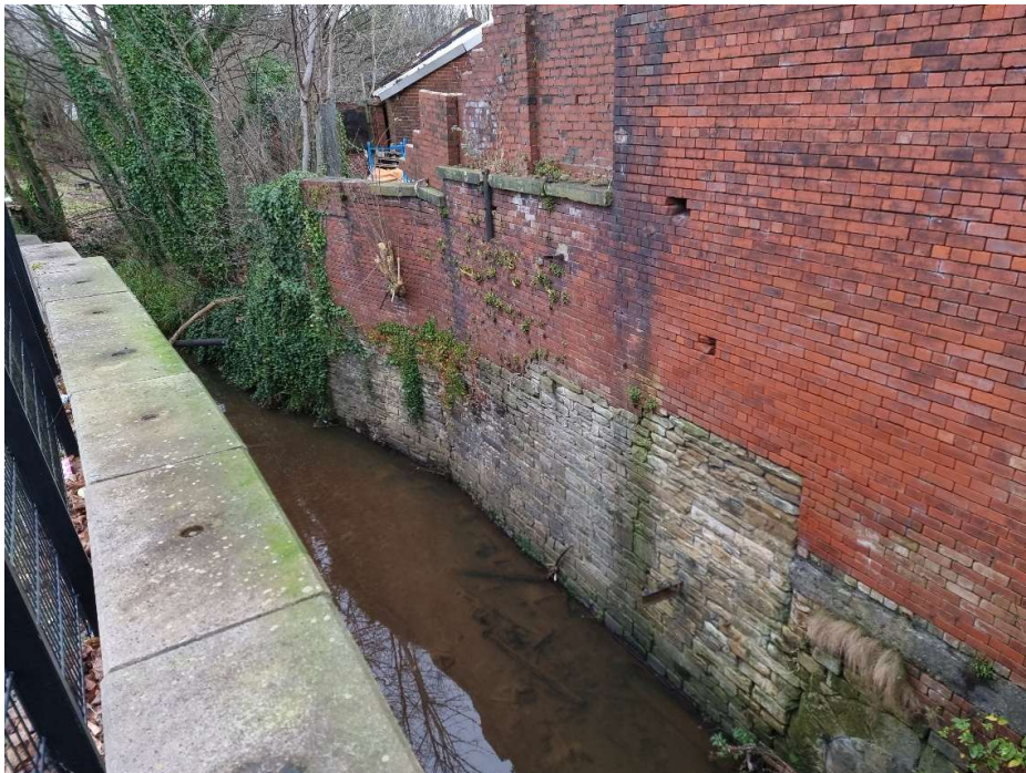
Photograph 2 – South East elevation of 2 storey mill with Sudden Brook running adjacent to the Southern boundary of the application site.
