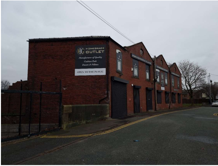
Photograph 1 – South East elevation of two storey mill, the proposed apartments are to be located on the ground floor of this section of the building – elevation approximately 5.3m above the Sudden Brook
