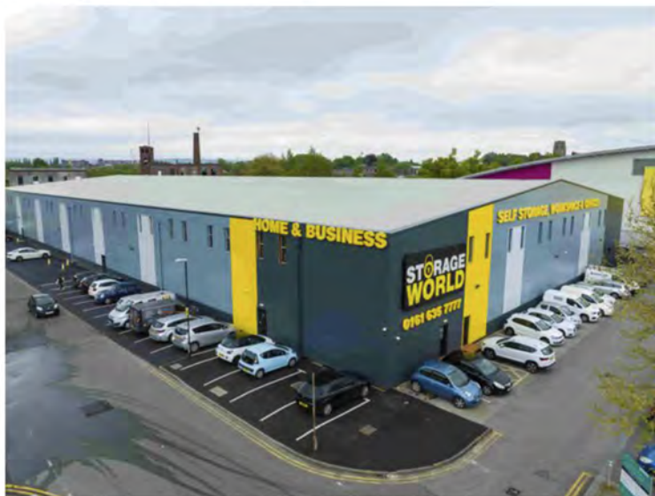
Storage World from Old Hall Street
