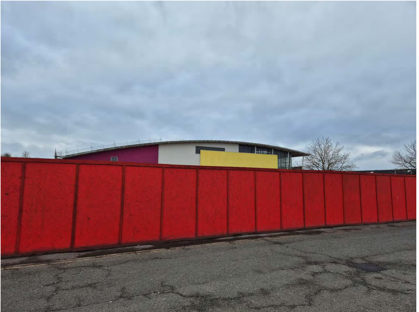
Plate 2: Hoarding bounding the Site, looking broadly south/south-east
