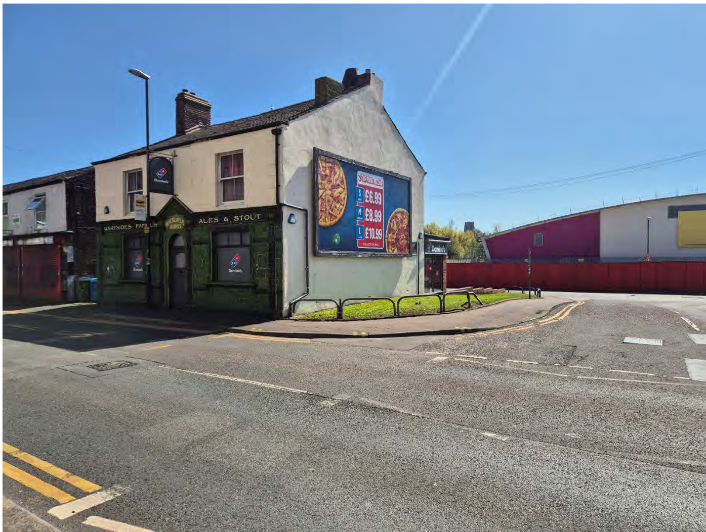
Plate 29: View of the former public house, with Site visible to the rear, looking south/south-east
