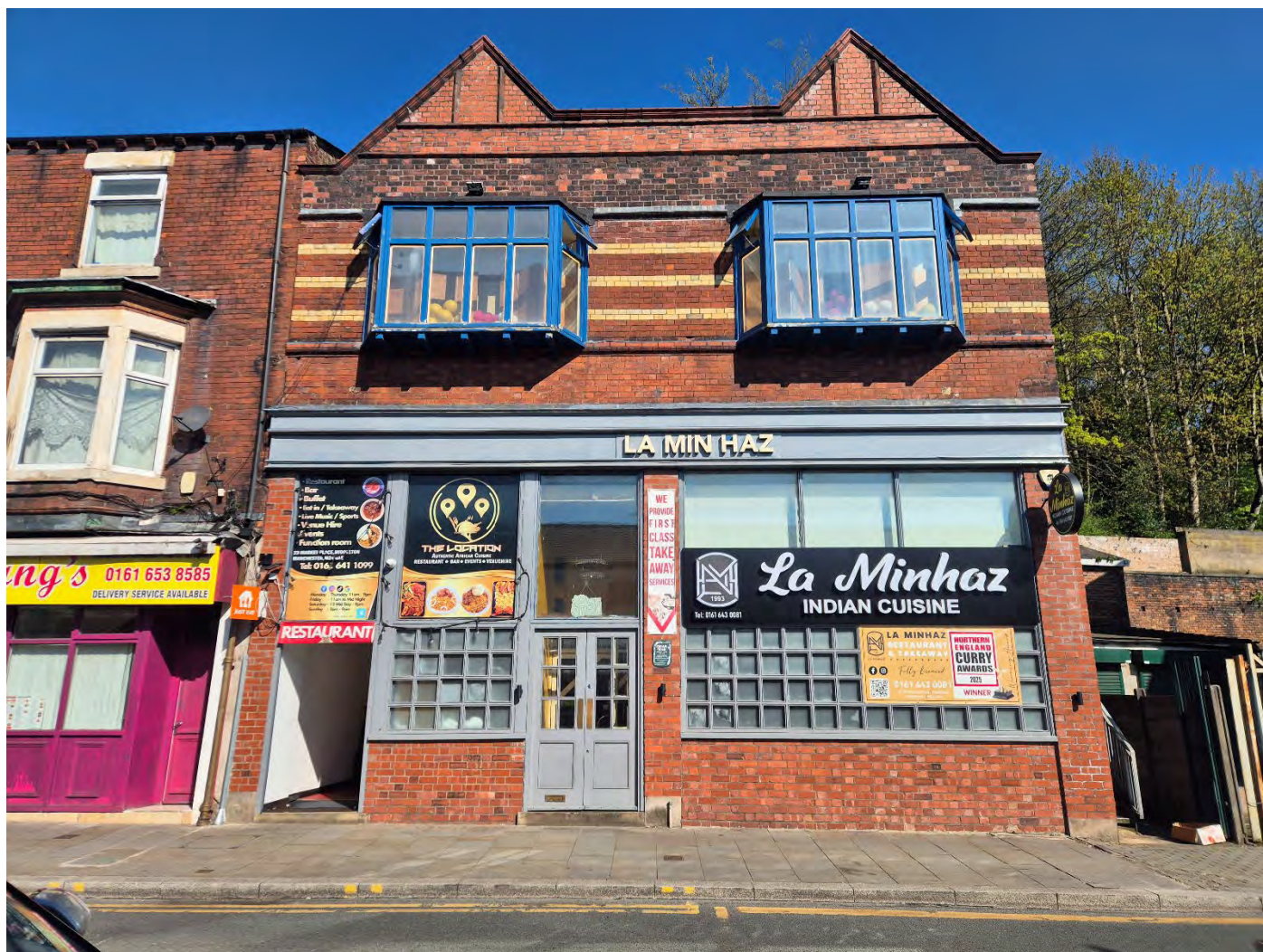
Plate 30: View of the building looking north from Market Place, looking north
