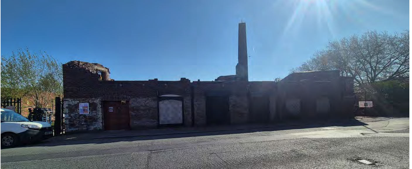
Plate 27: View of Lodge Mill following the fire, looking east
