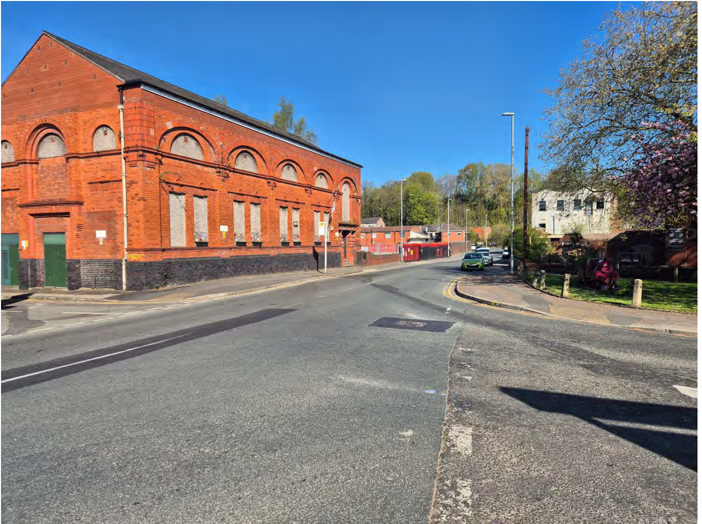
Plate 21: Key View looking north along Townley Street
