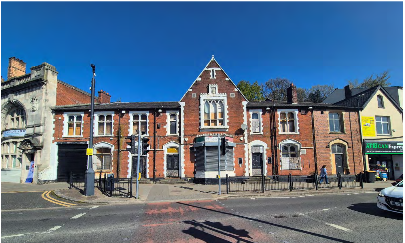
Plate 24: Principal elevation of the former Police Station, looking north
