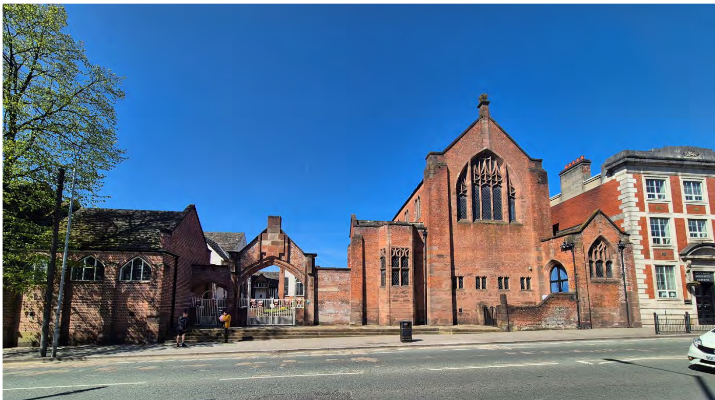
Plate 17: Loomshop in left of frame, methodist church in centre and right of the frame
