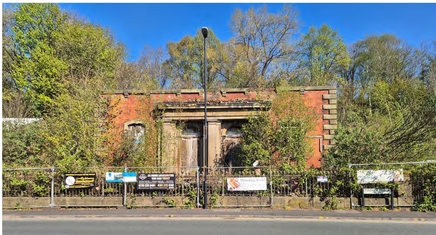
Plate 11: View of the former chapel, showing the partial demolished front elevation of the building, looking north
