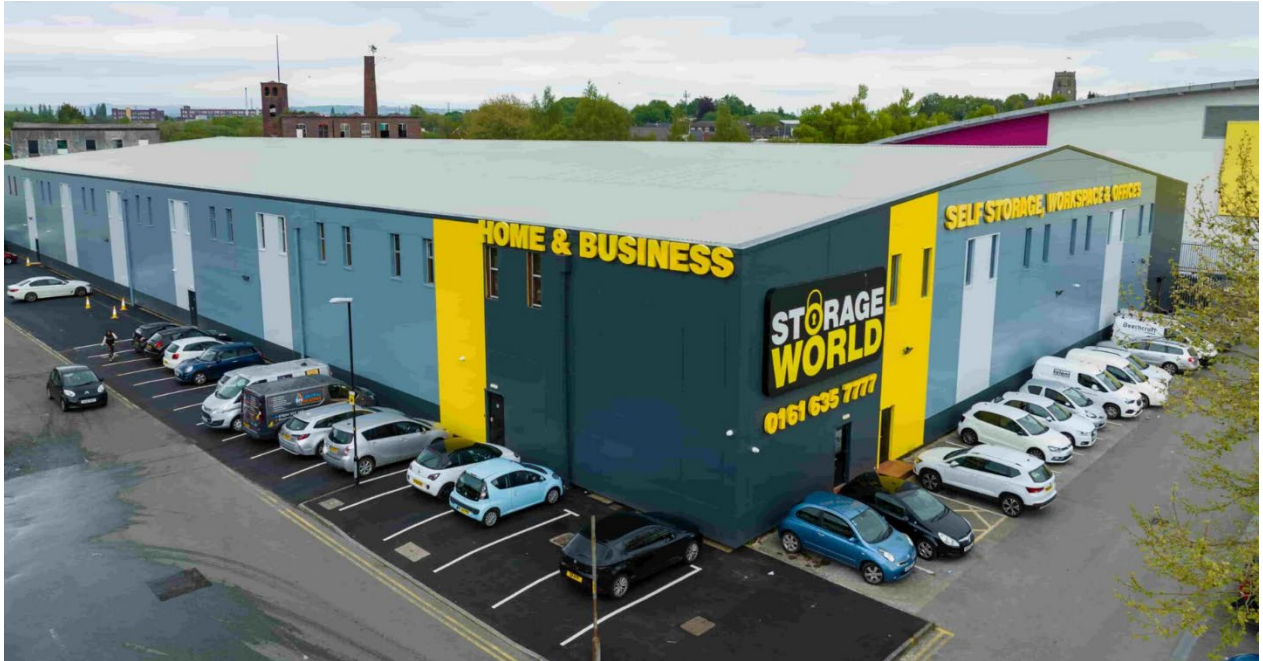
Photograph of Storage World facility in Middleton prior to fire.
