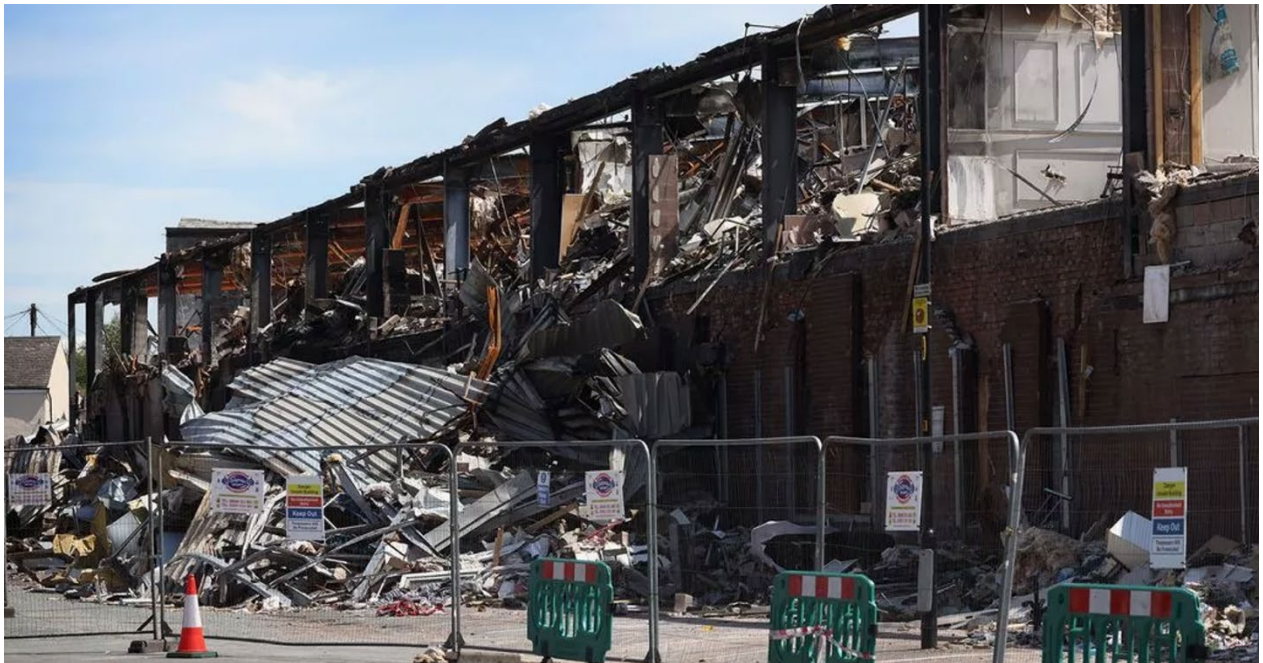
Photograph of Storage World facility in Middleton post-fire (taken from Sean Hansford, Manchester Evening News, 2025)
