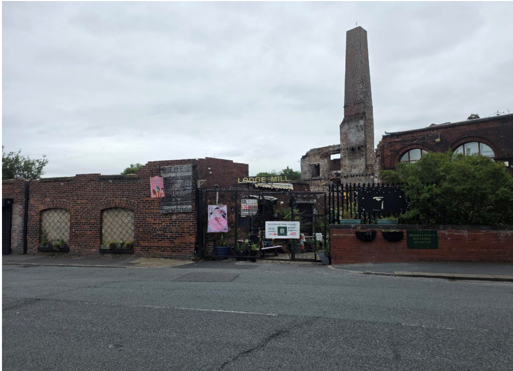
Lodge Mill opposite site on Townley Street following April 2026 fire
