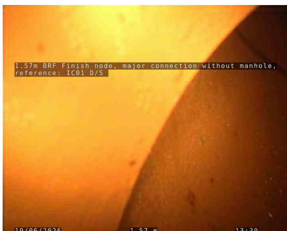
5, 00:00:48, 1.57 m Finish node, major connection without manhole, reference: IC01 D/S, JOINS NEW LINE
