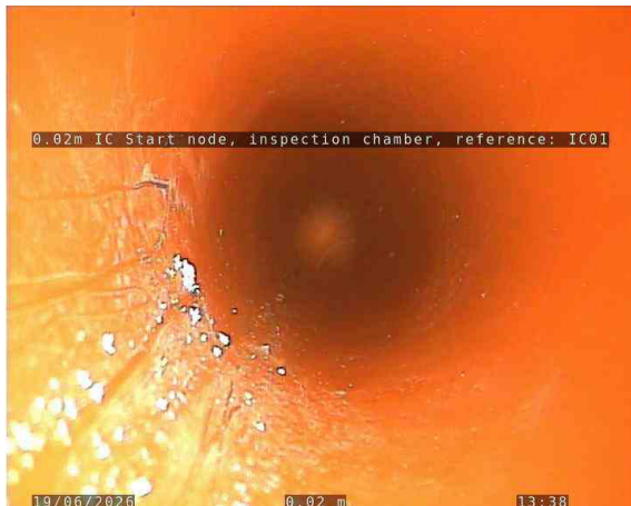
1, 00:00:01, 0.02 m Start node, inspection chamber, reference: IC01
