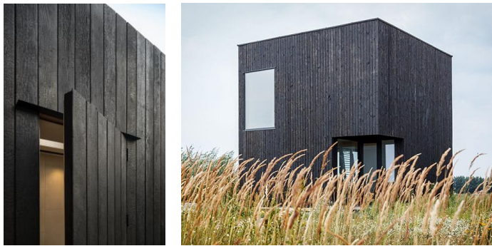
charred timber cladding
