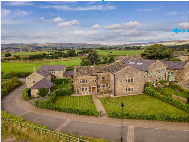
Birchinley Manor south-facing elevation
