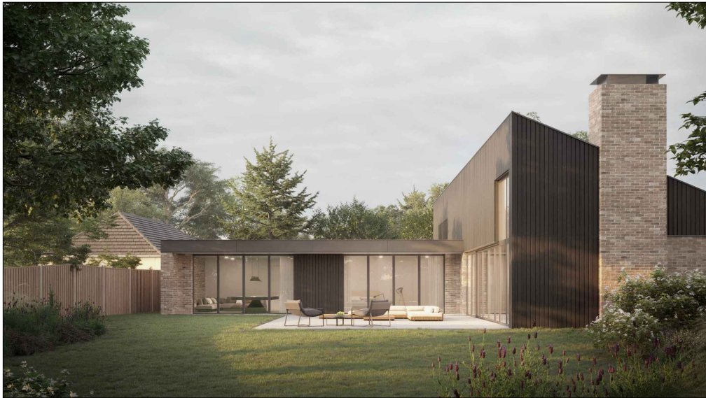
charred timber + brick (light-buff)
