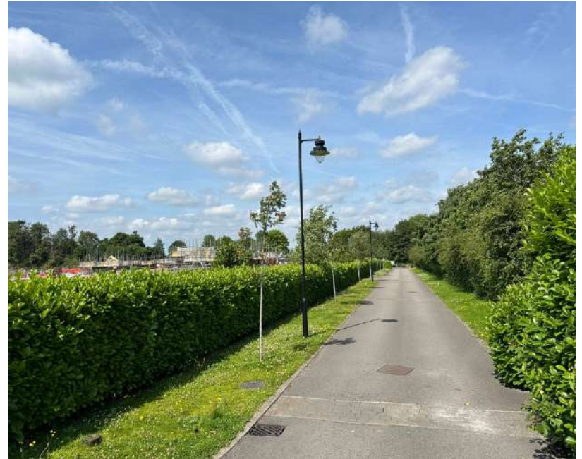
Figure 3.16: View of the neighbouring development under construction (July 2024)
