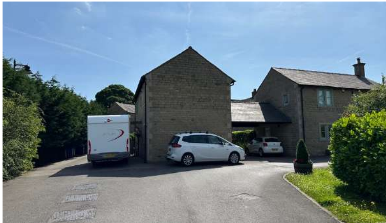
Figure 4.11: View to Birchinley Hall (2024)
