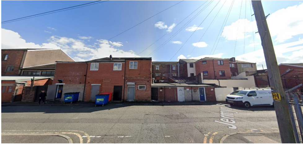
Figure 3Rear servicing access from Jermyn Street
