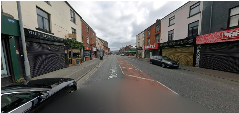
Figure 1 View of Yorkshire Street commercial frontage
