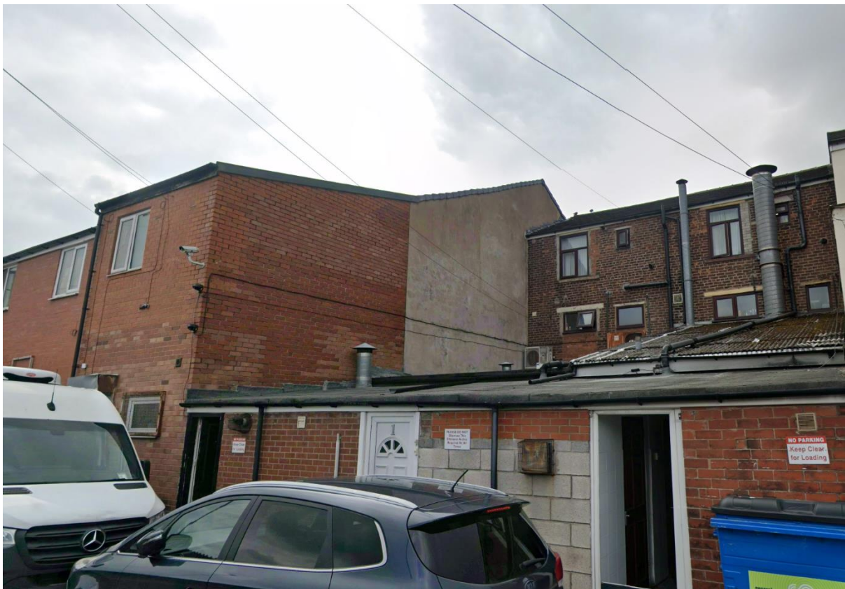
Figure 8 Existing commercial servicing and extraction equipment within the surrounding area
