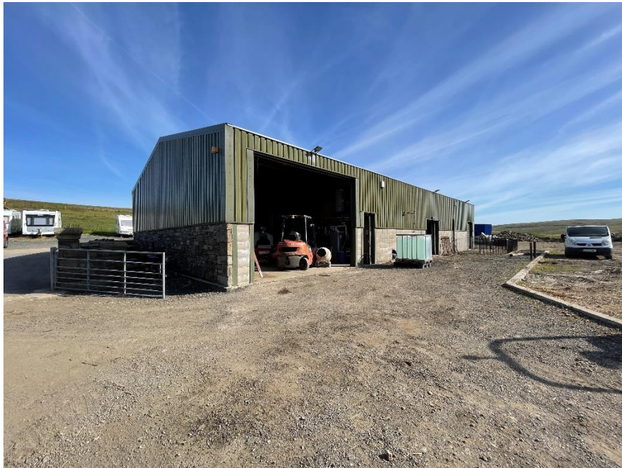
Photo 2 - Agricultural Building view from northwest
