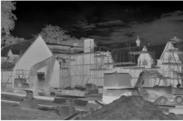
Thermal camera coverage at end of survey
