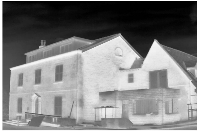
Thermal camera coverage at end of survey
