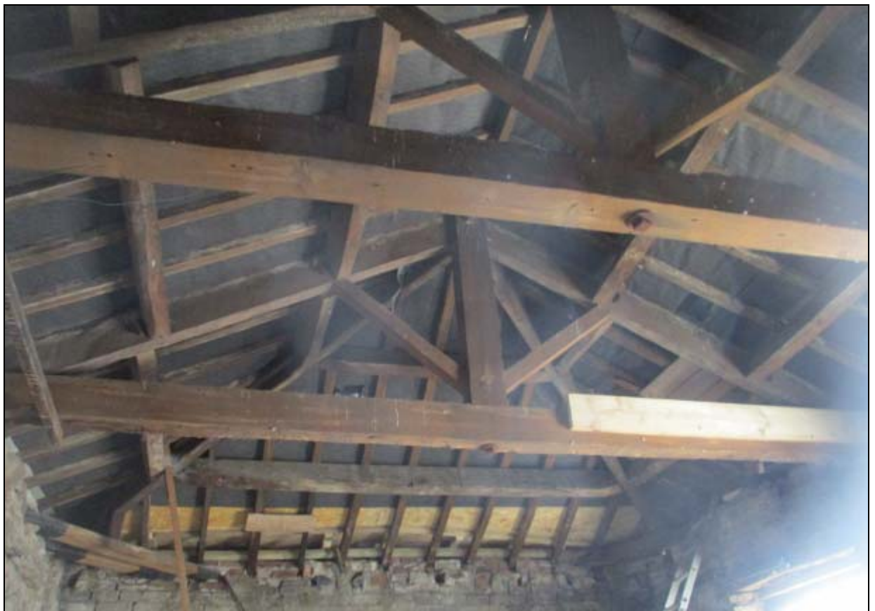
Kingpost roof trusses in rear wing
