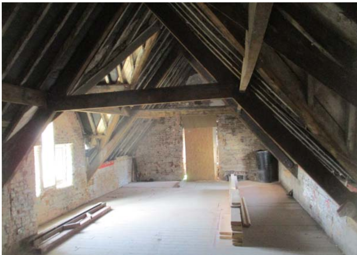
Trusses in room at far end of rear wing
