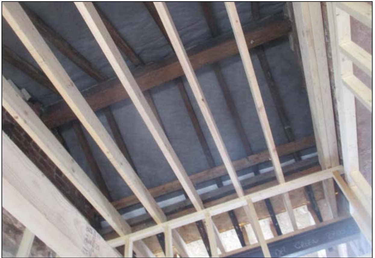
Exposed probably replaced purlins on first floor of circa 1814 main block
