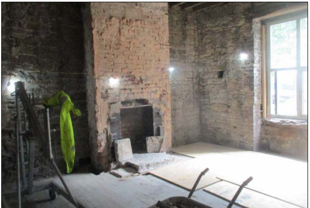
Ground floor front right room showing chimneybreast
