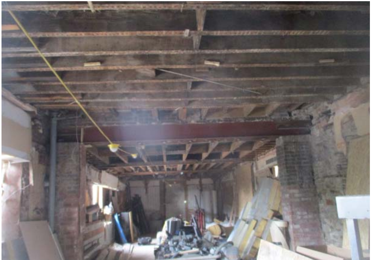
View into rear wing showing late 20 th century steel beam and replacement joists
