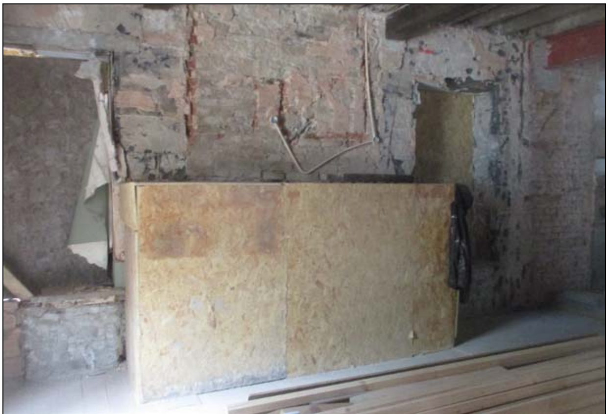
Ground floor front left room, with existing fireplace protected
