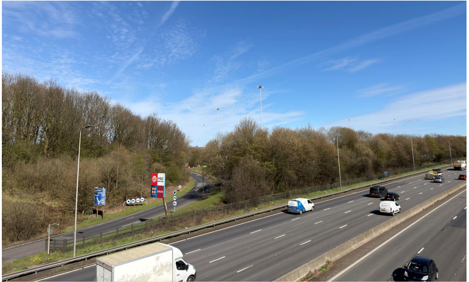
The M62 motorway, with dense tree planting on either side, is located between the Birch Village Business Park and the Site. As a result, the Site is physically and visually divorced from the conservation area
